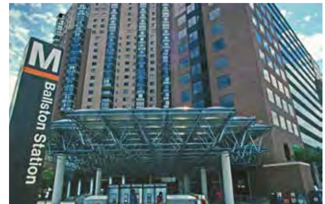
Ballston Station. An early example of high density air rights development over the Metro Station.
