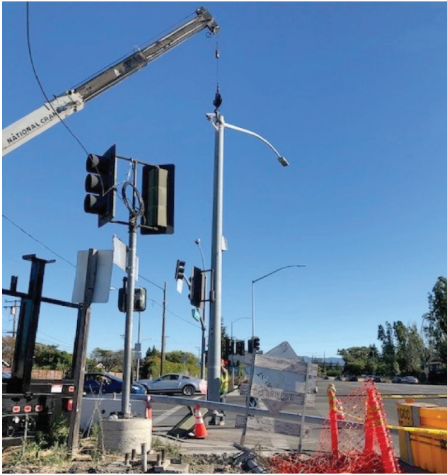
◀ Temporary signal light installation at Ross Drive
