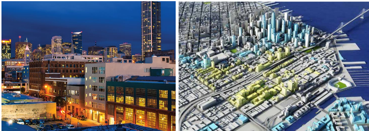
FIGURE VI-5. CENTRAL SOMA TODAY (LEFT) AND CENTRAL SOMA 3-D MODEL OF POTENTIAL DEVELOPMENT (RIGHT)
