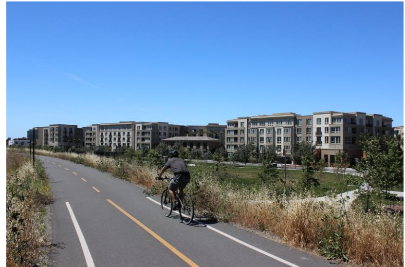
Example of TOD promoting multi-modal lifestyle at River View adjacent to VTA's River Oaks Station
