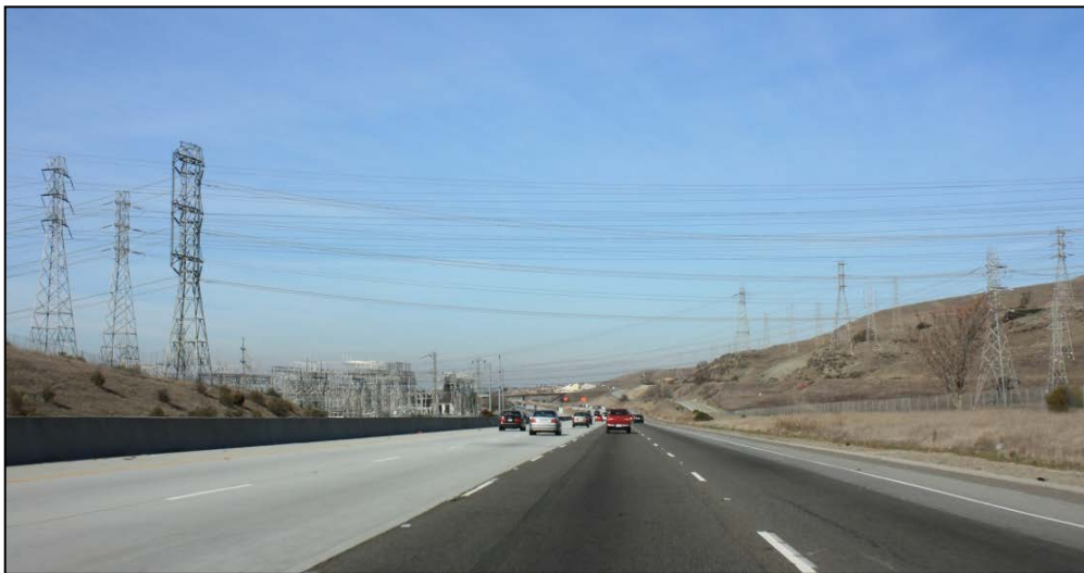
Exhibit F. Northbound US 101 north of Bailey Avenue in southern San Jose. The PG&E Metcalf Substation is just west (left) of the southbound lanes.
