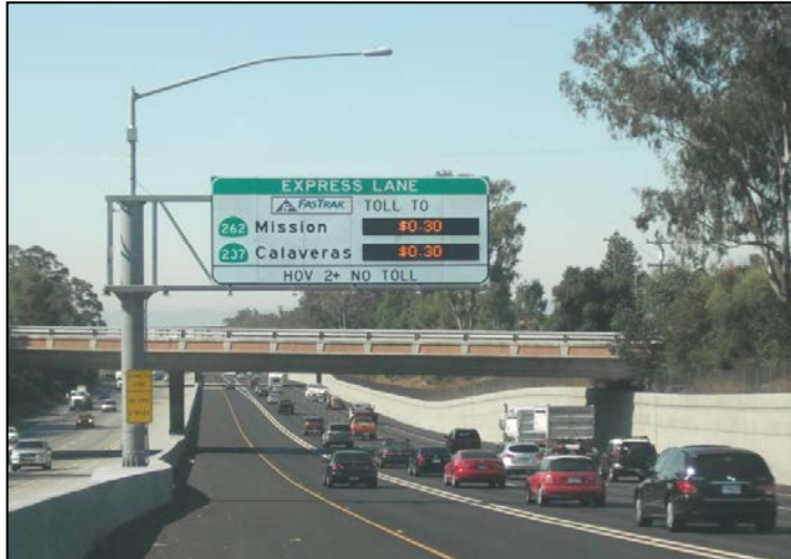
Exhibit M. Representative view of an entrance/toll sign with messaging (from I-680 southbound express lanes in Fremont)
