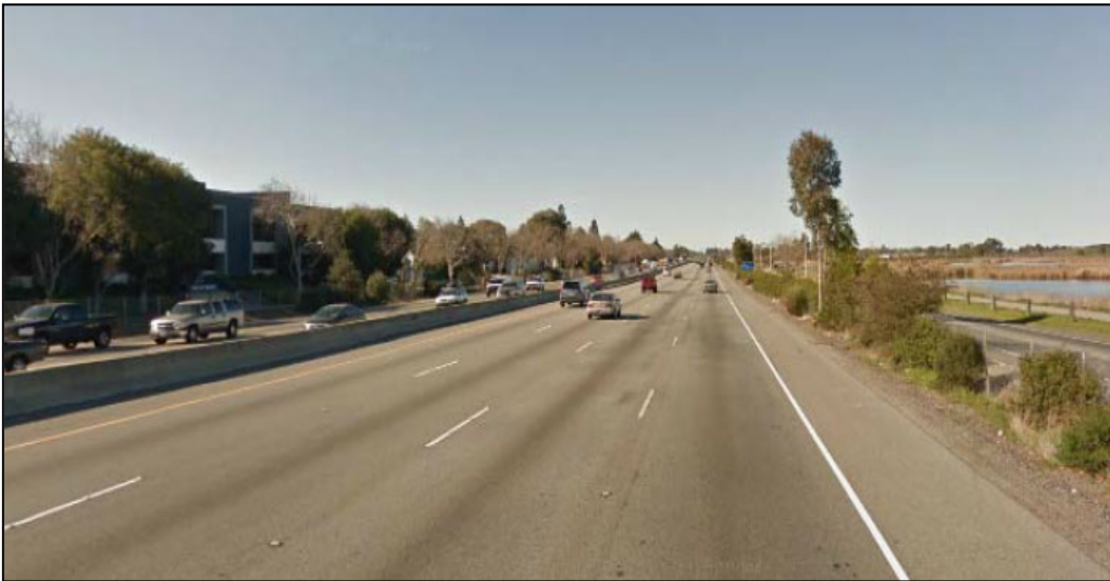
Exhibit K. Northbound US 101 north of San Antonio Road in Palo Alto; Palo Alto Baylands Park is to the east (right)
