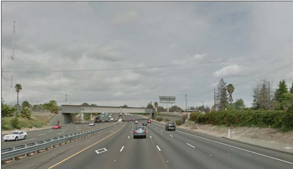
Exhibit H. Northbound US 101 just north of McKee Road in San Jose. A railroad overcrossing and overhead utility lines can be seen in the distance.
