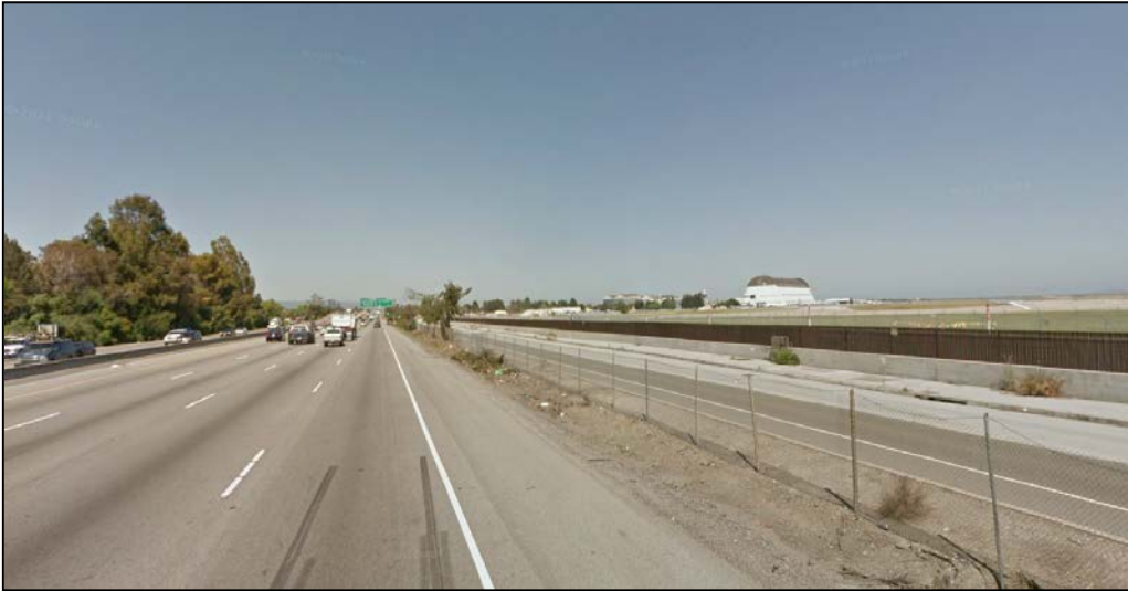
Exhibit J. Northbound US 101 south of Ellis Street interchange near the Sunnyvale/ Mountain View border. Moffett Federal Airfield borders US 101 to the east (right).
