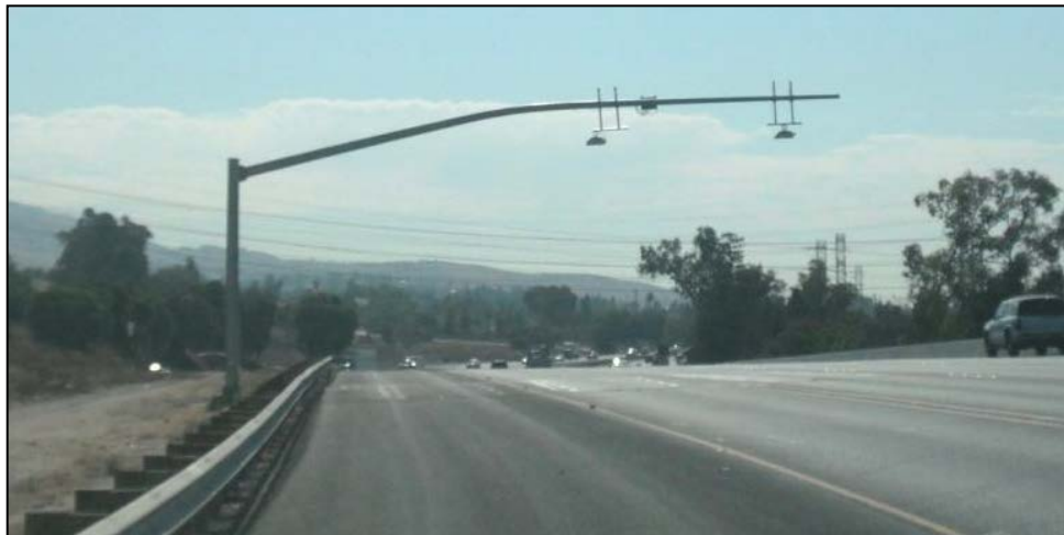
Exhibit P. Representative view of a toll structure (viewed from I-680 southbound express lanes in Fremont)
