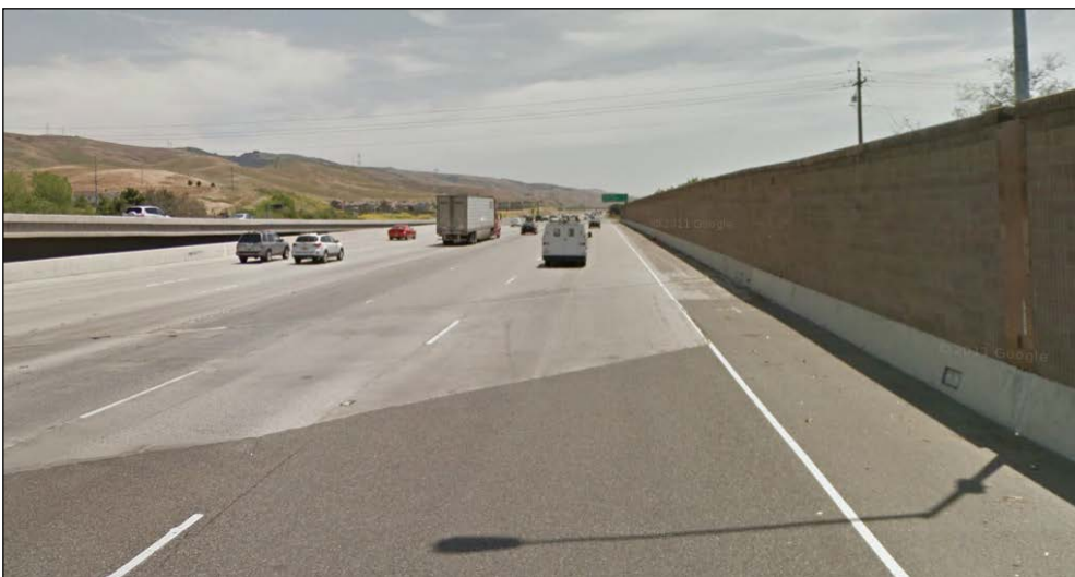
Exhibit D. Southbound US 101 south of SR 85 interchange in southern San Jose, with a sound wall on the west side (right) of the freeway.
