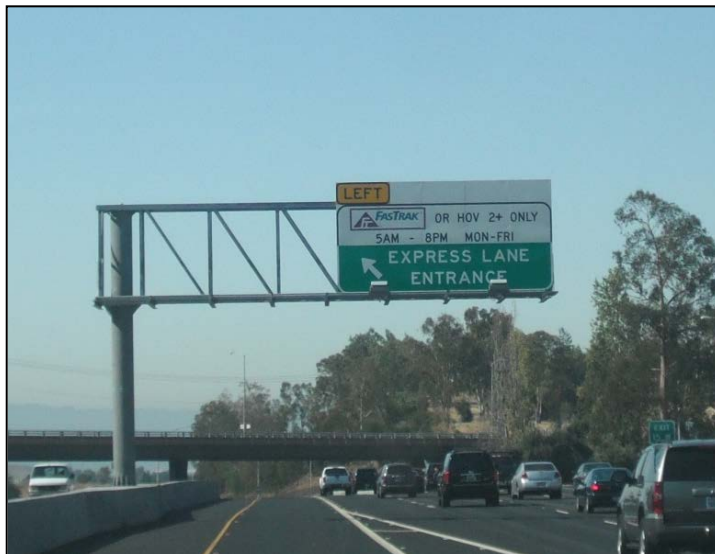
Exhibit N. Representative view of an express lane entrance sign (from I-680 southbound express lanes in Fremont)
