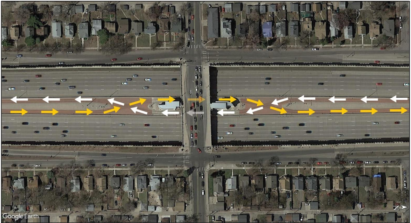
Figure 9 Aerial View of Median Crossover Platform Station at I-35W/46th Street
