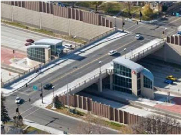
46th: Existing BRT Station
