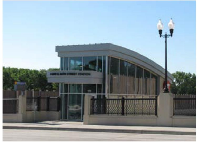
46th: Entrance to BRT Station
