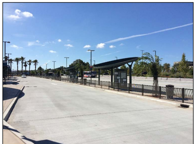
Completed Bus Shelter and Bus Bay at the Eastridge Transit Center
