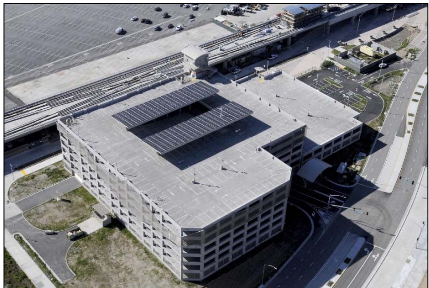
Berryessa Station Parking Garage Solar Panel System
