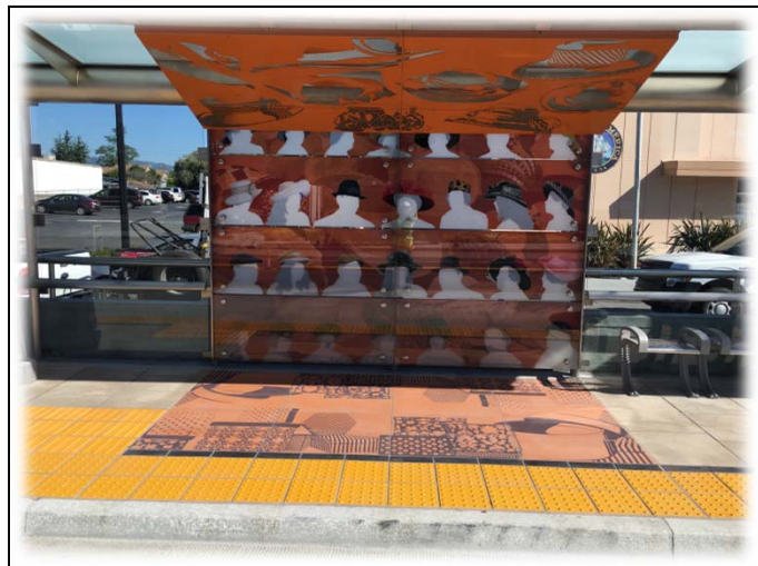
BRT Station shelter - Jackson St Eastbound Station
