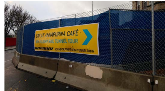
Advertisement for local business during construction of Capitol Hill Light Rail Station – Sound Transit
