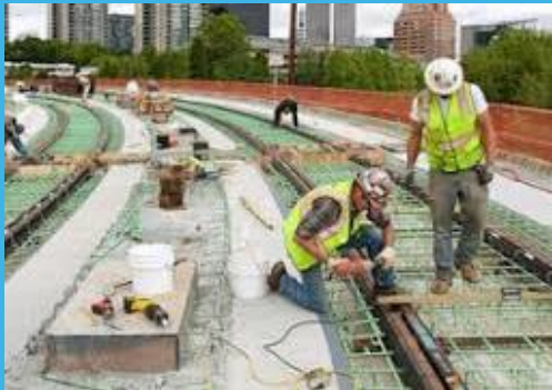
Light Rail Construction
