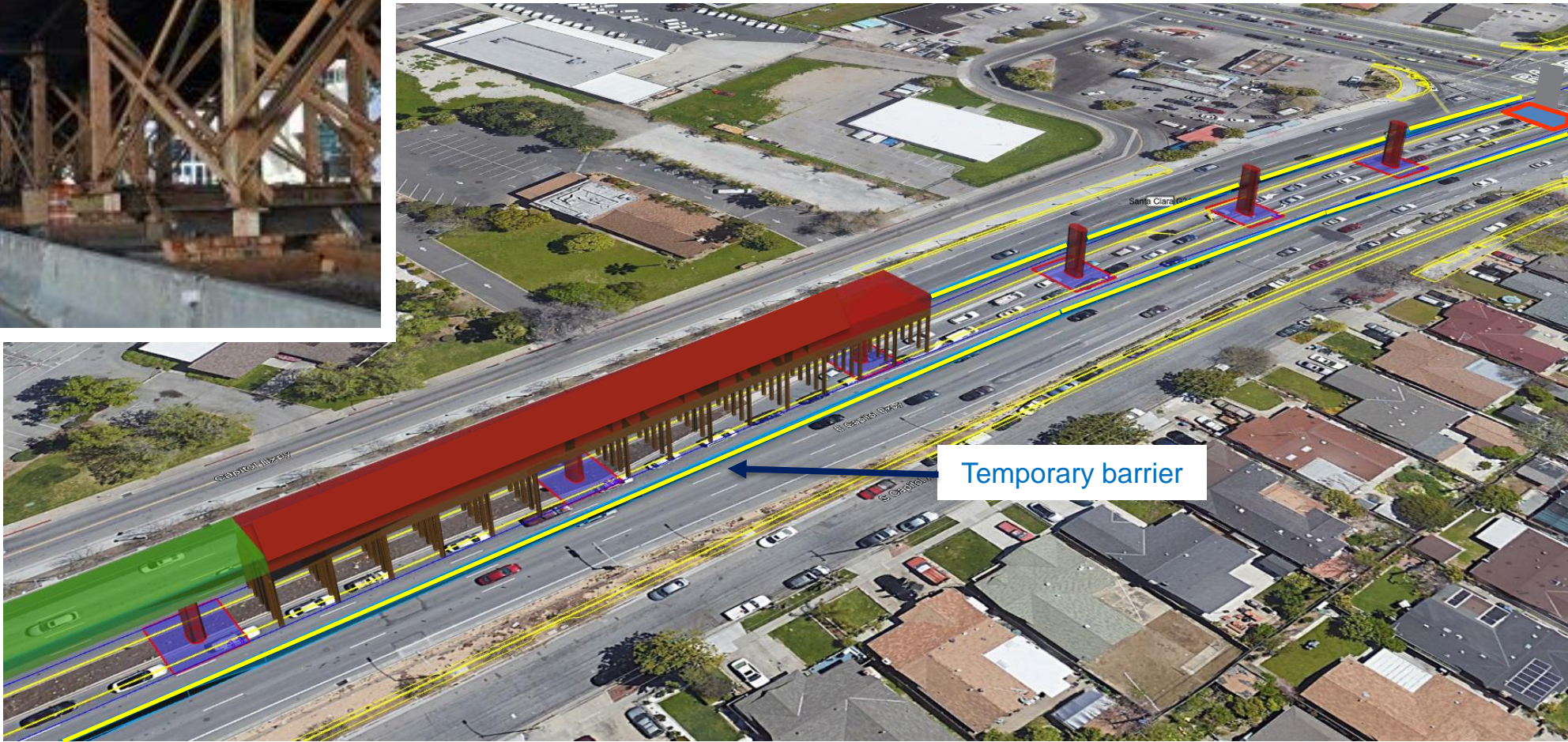
Concrete barrier placed at beginning of construction to protect open footing, pile driving, falsework, etc.
