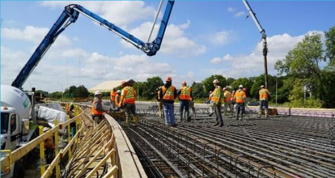
Bridge Steel and Concrete
