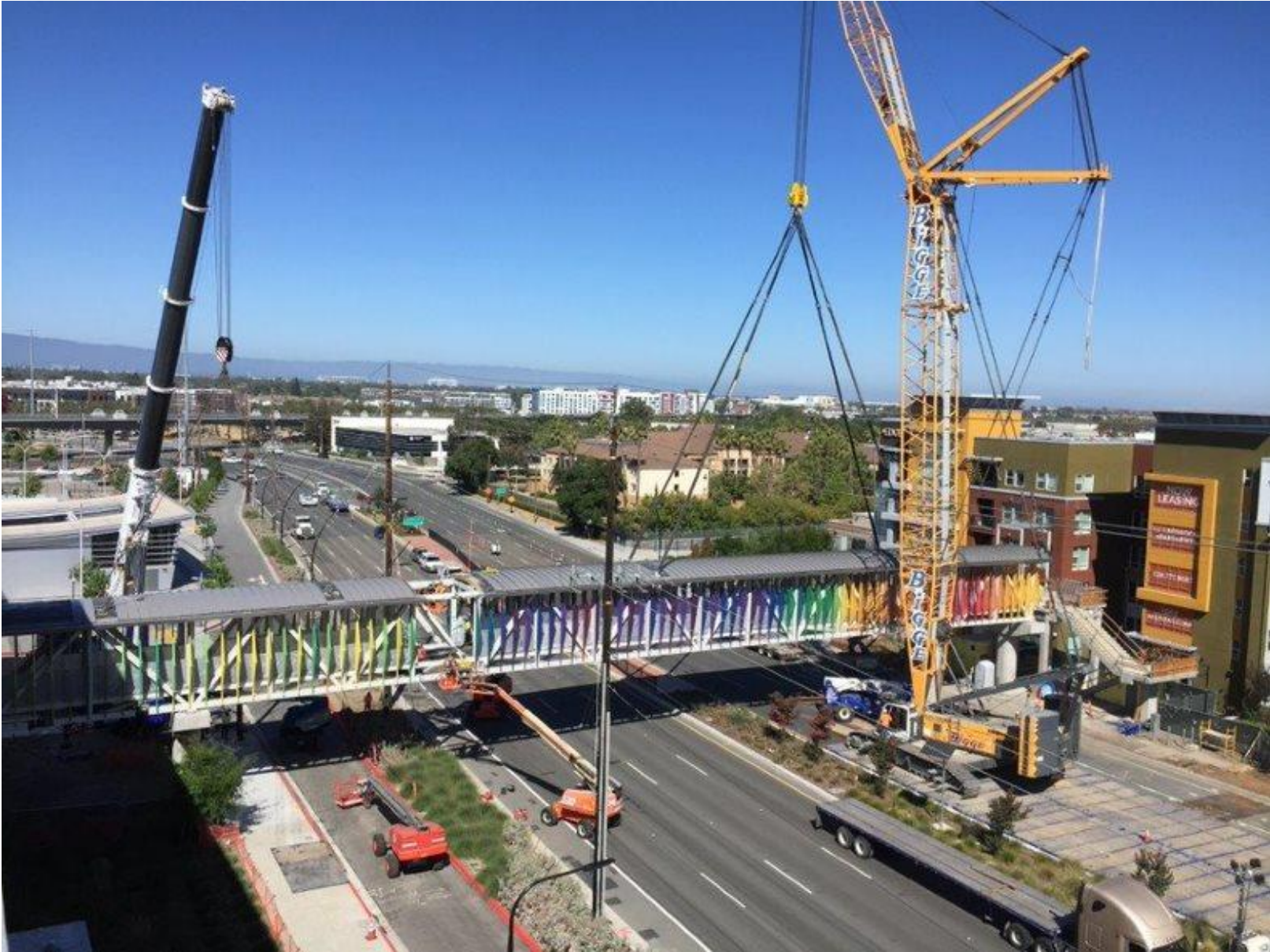
Montague Pedestrian Overcrossing in July 2020
