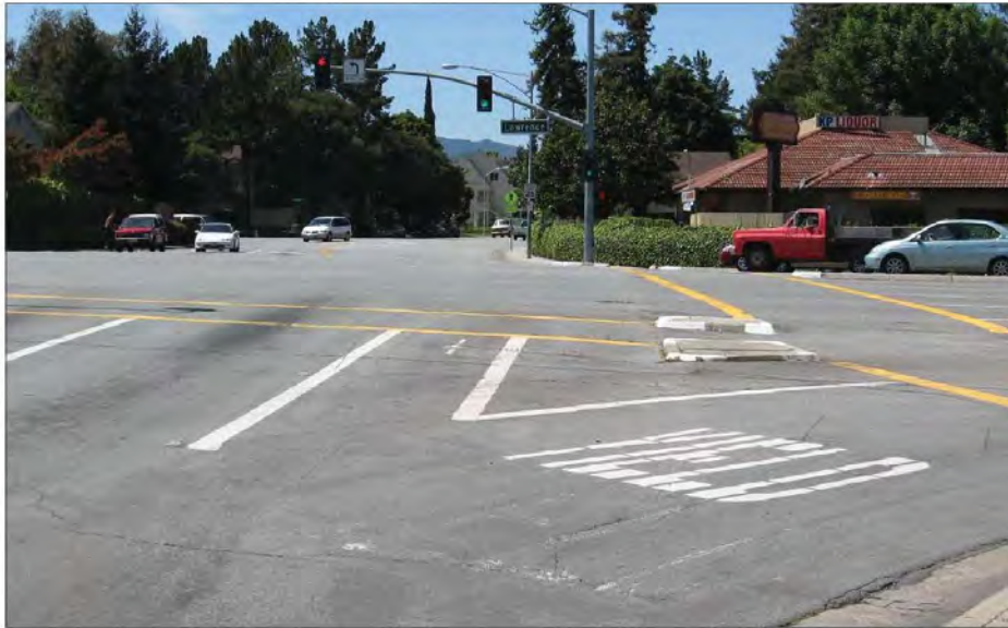
a. View of an example bike slot facing west at Lawrence Expressway and Cabrillo Avenue in the City of Santa Clara.
