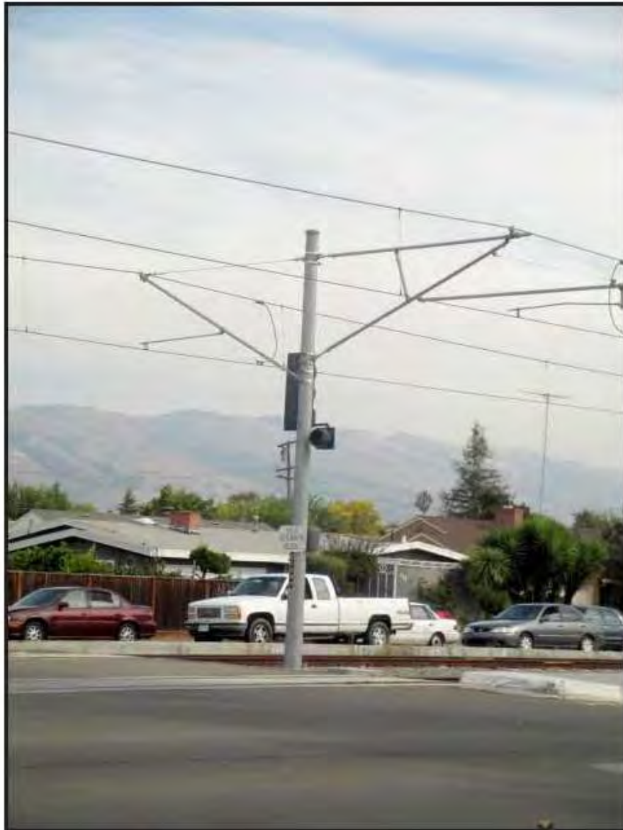
Figure 4 Overhead Contact System at Alum Rock Station
