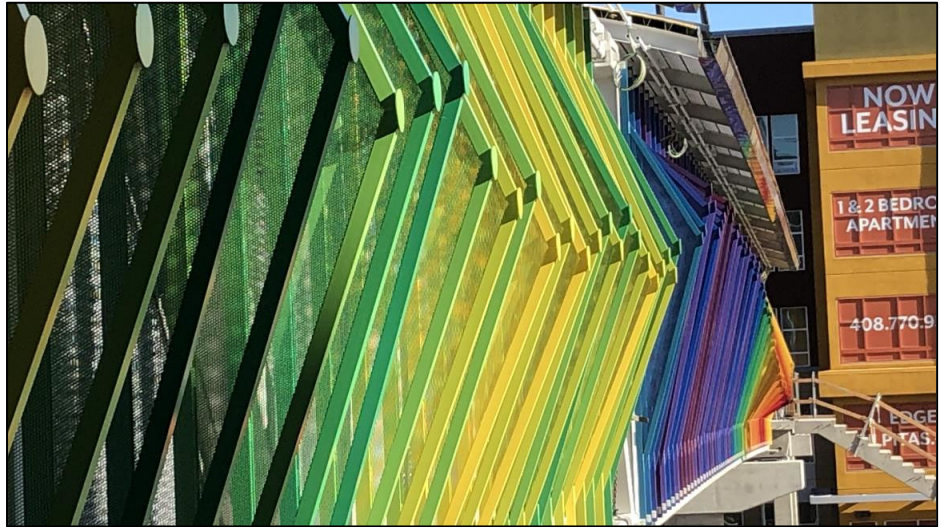
Montague Pedestrian Overcrossing Bridge
