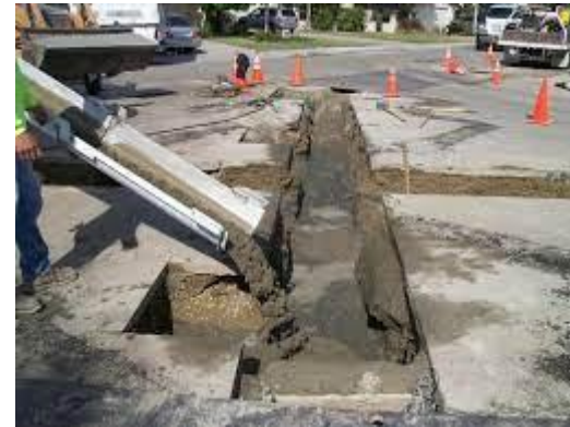
Backfill Trench
