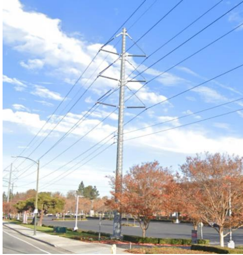
Overhead Wires Installed
