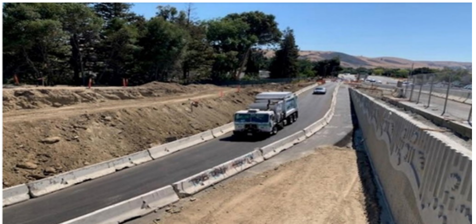
New retaining wall west of the northbound on-ramp toward US 101 off Blossom Hill Road.
