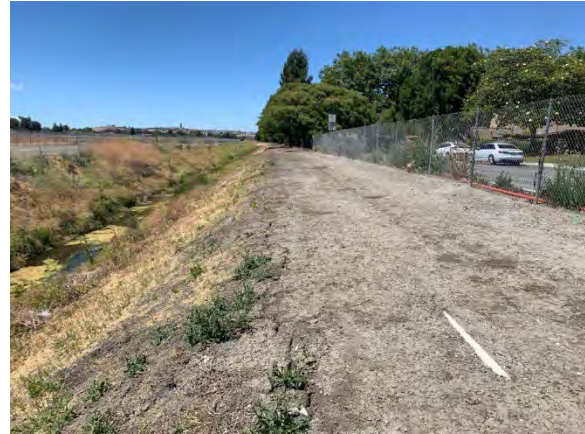
Photo 5. The Valley Water access road and Canoas Creek channel to the north of State Route 85 (view to the north).
