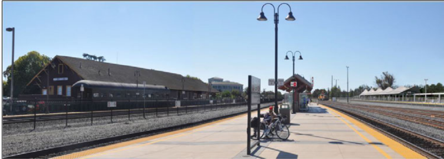
Figure 5-22: Existing View (top) and Simulated View (bottom) of the Santa Clara Depot (left) looking northwest from the Caltrain station platform, showing the proposed at-grade tracks and Santa Clara Depot platform (far right) under both the Single- and Twin Bore Options.
