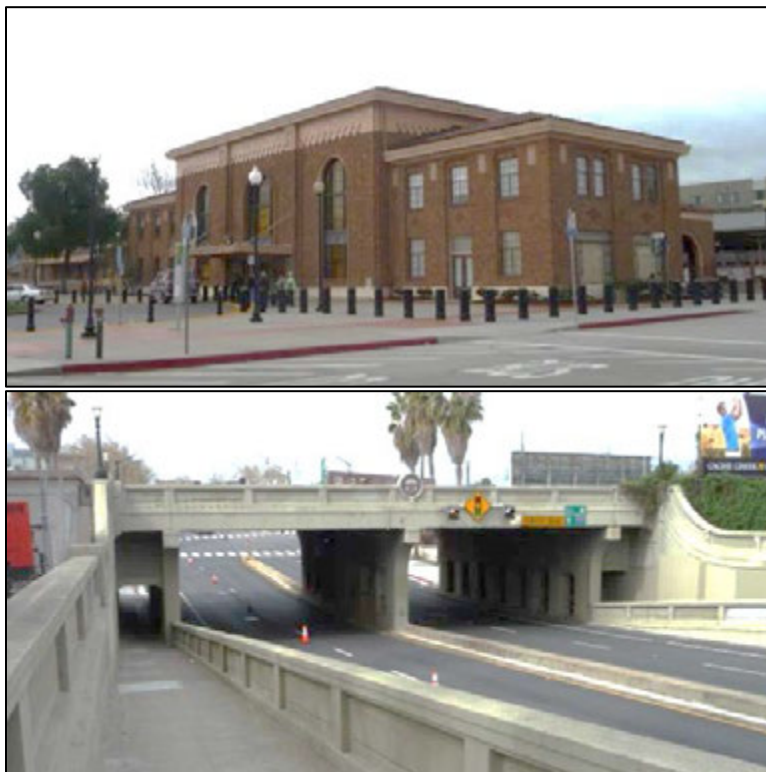
Photographs 4-18 and 4-19: Cahill/Diridon Station (top) and Santa Clara/Alameda Underpass (bottom).
