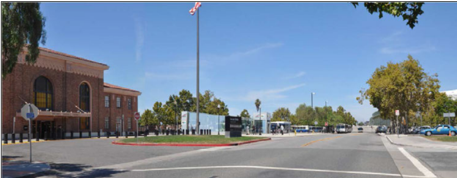
Figure 5-20: Existing View (top) and Simulated View (bottom) of the Diridon Station South Option (Twin-Bore Option) E1 station entrance option looking north along Cahill Street showing the Southern Pacific Depot (left).
