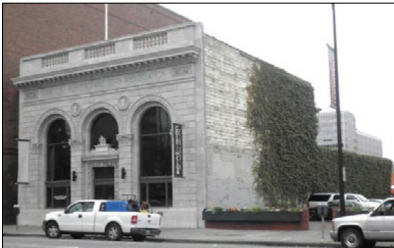
Photograph 4-12: San Jose Building and Loan (81 West Santa Clara Street).
