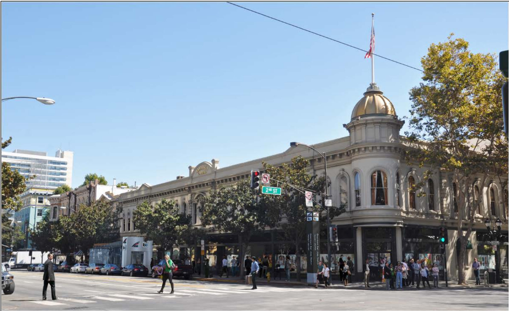
Figure 5-8: San Jose Downtown Commercial District, Existing View (top) and Simulated View (bottom) of the Downtown San Jose Station—West Option (Twin-Bore Option) E6 entrance option. Views are looking southeast along Santa Clara Street showing South 3 rd Street (far right) and historic district contributor (Map Reference E-13, middle right, and Map Reference E-14, middle left).
