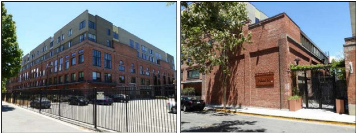
Photographs 4-24 and 4-25: Del Monte/Cal Pak Plant #51 at 88 Bush Street.
