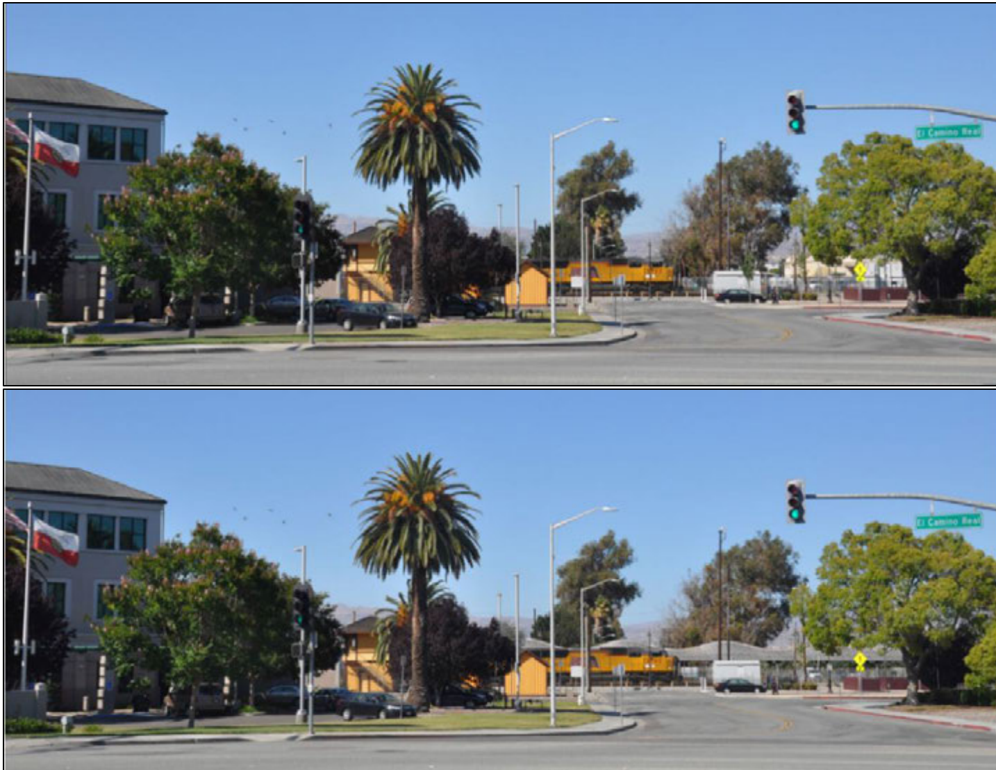
Figure 5-24: Existing View (top) and Simulated View (bottom) looking north from the intersection of El Camino Real and Railroad Avenue toward the Control Tower, Maintenance of Way Speeder Shed, and Maintenance of Way Section Tool House (center right) and showing the proposed Santa Clara Depot platform in background for both the Single- and Twin-Bore Options.
