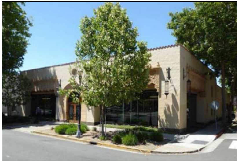
Photograph 4-26: Commercial building at 865 The Alameda.
