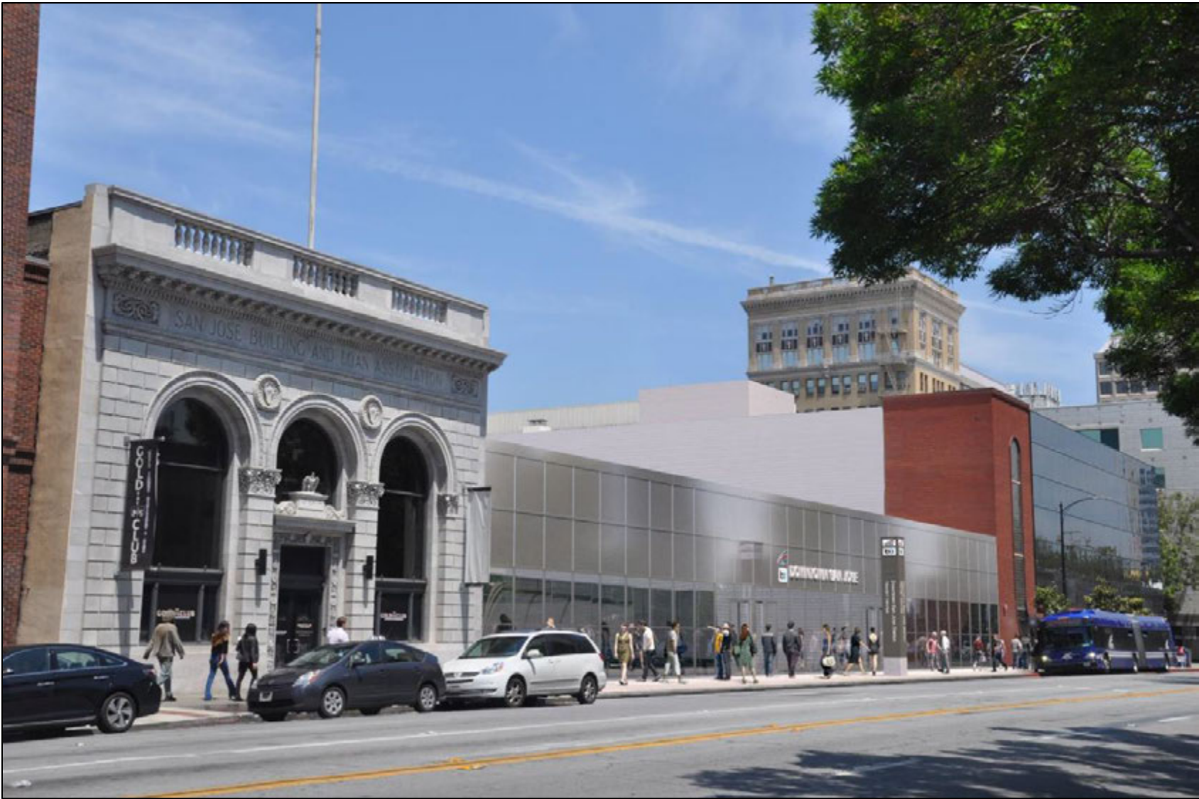
Figure 5-13: 81 West Santa Clara Street, Existing View (top) and Simulated View (bottom) of Downtown San Jose Station—West Option (Twin-Bore Tunnel Alignment) E3 entrance option, looking northwest from West Santa Clara Street.
