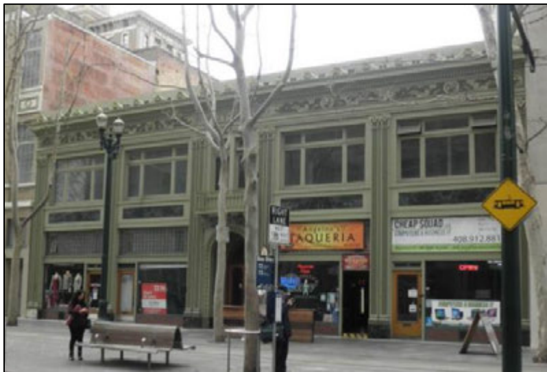
Photograph 4-9: Detail of west side of the Realty Building's main façade (19 North 2 nd Street).
