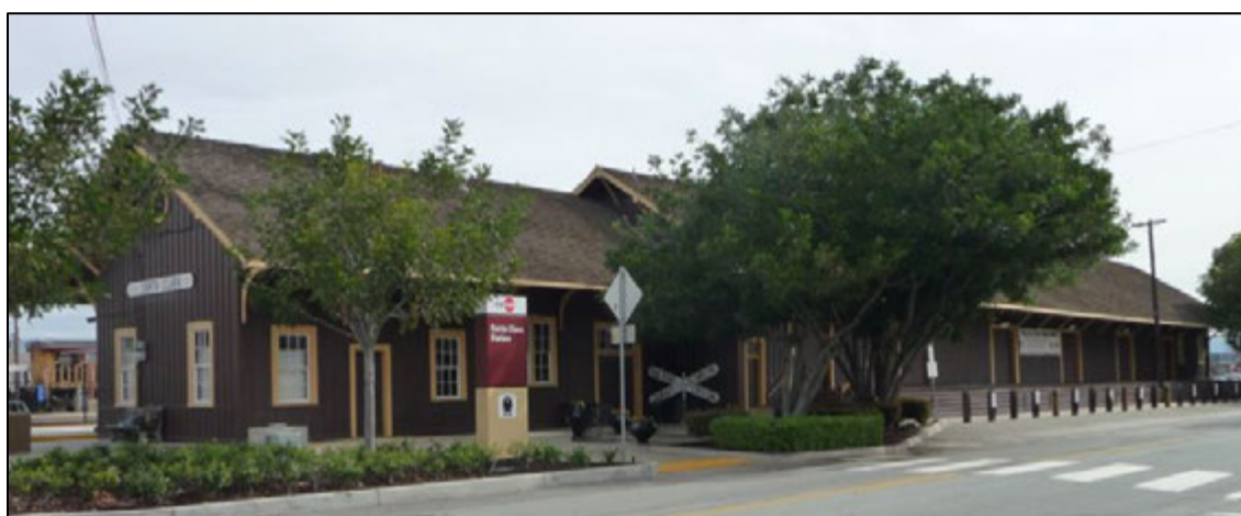
Photograph 4-27: Santa Clara Station (1 Railroad Avenue).
