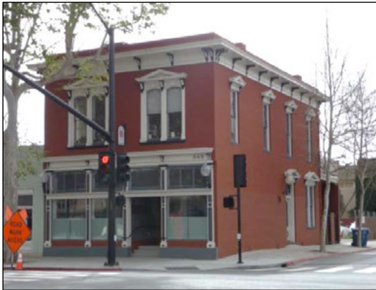
Photograph 4-20: Commercial building at 848 The Alameda.
