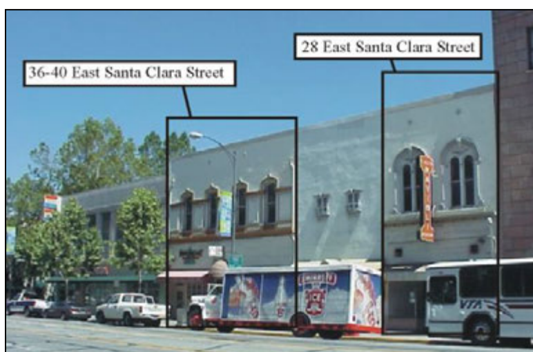
Photograph 4-5: Contributors to the San Jose Commercial Historic District, 36-40 East Santa Clara Street and 28 East Santa Clara Street. The unlabeled building in-between is a noncontributory.
