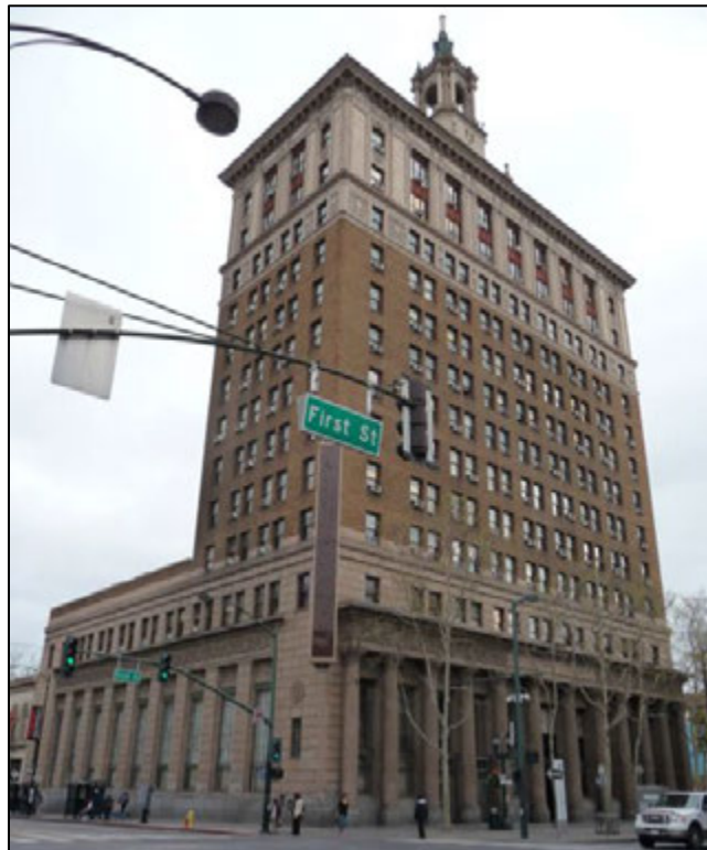
Photograph 4-8: The Bank of America building at 8-14 South 1 st Street.
