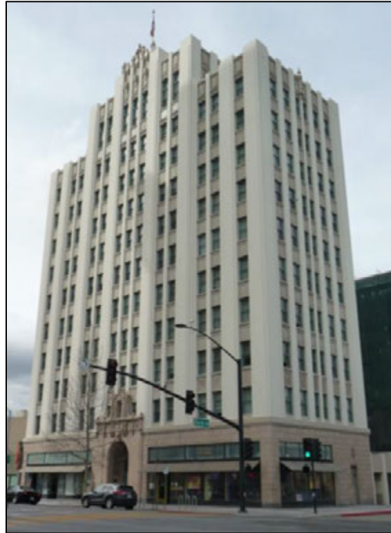
Photograph 4-4: Vintage Towers (Medico Dental Building) at 227-247 East Santa Clara Street.
