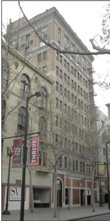
Photograph 4-10: The Commercial Building (22 North 1 st Street).
