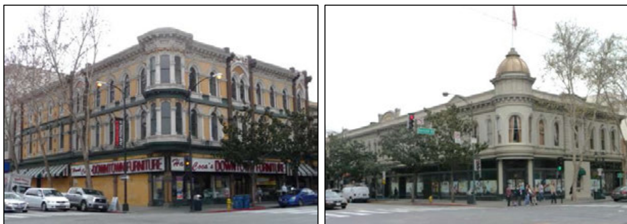
Photographs 4-6 and 4-7: Odd Fellows Building (96 East Santa Clara Street, shown left) and commercial building at 52 East Santa Clara Street (right).
