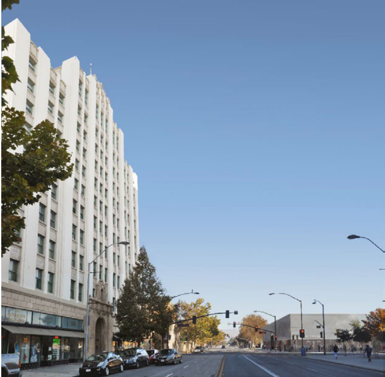
Figure 5-4: 227-247 East Santa Clara Street, Existing View (top) and Simulated View (bottom) of the Downtown San Jose Station – East Option (Single-Bore Tunnel Alignment) looking northeast along East Santa Clara Street toward 6 th Street .
