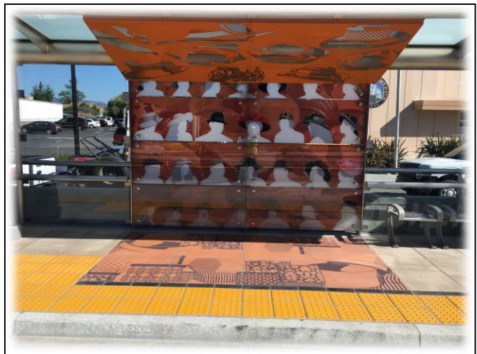
BRT Station shelter - Jackson Street Eastbound Station
