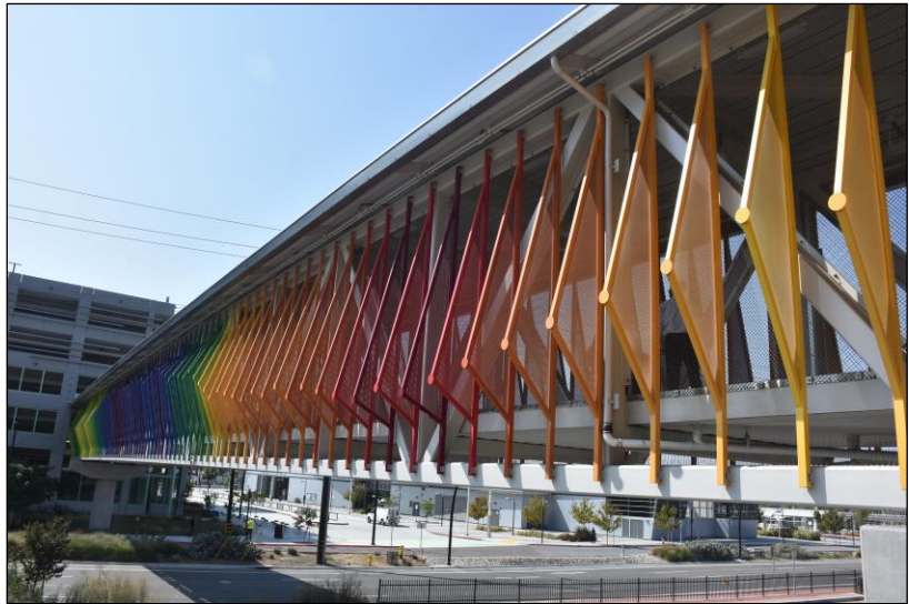
Montague Pedestrian Overcrossing Bridge
