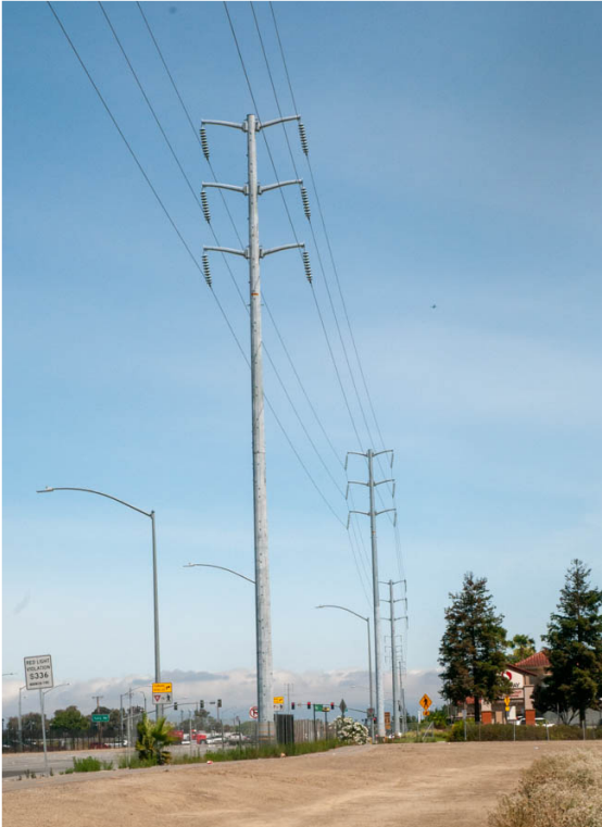
PG&E towers from the Thompson Creek Trail, looking north on Capitol Avenue.
