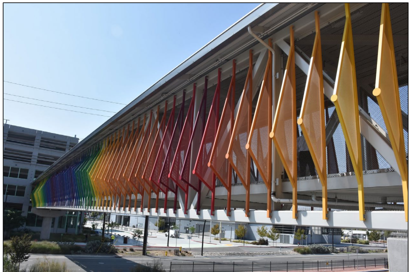
Montague Pedestrian Overcrossing Bridge
