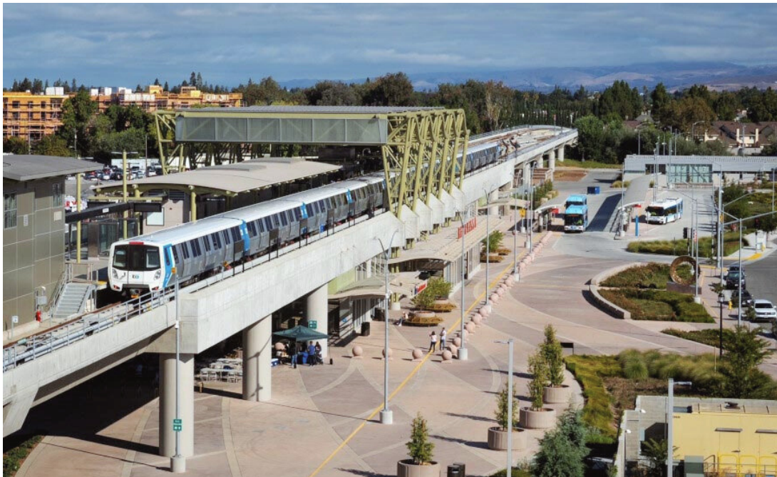
Elevated view of the Berryessa/North San José BART Station and Berryessa Transit Center.
