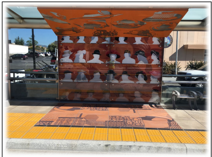
BRT Station shelter - Jackson Street Eastbound Station
