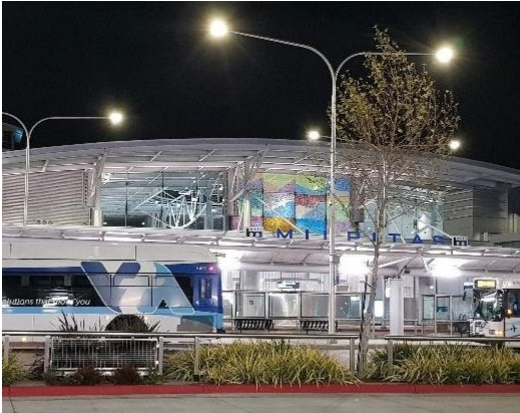
Milpitas BART Station
