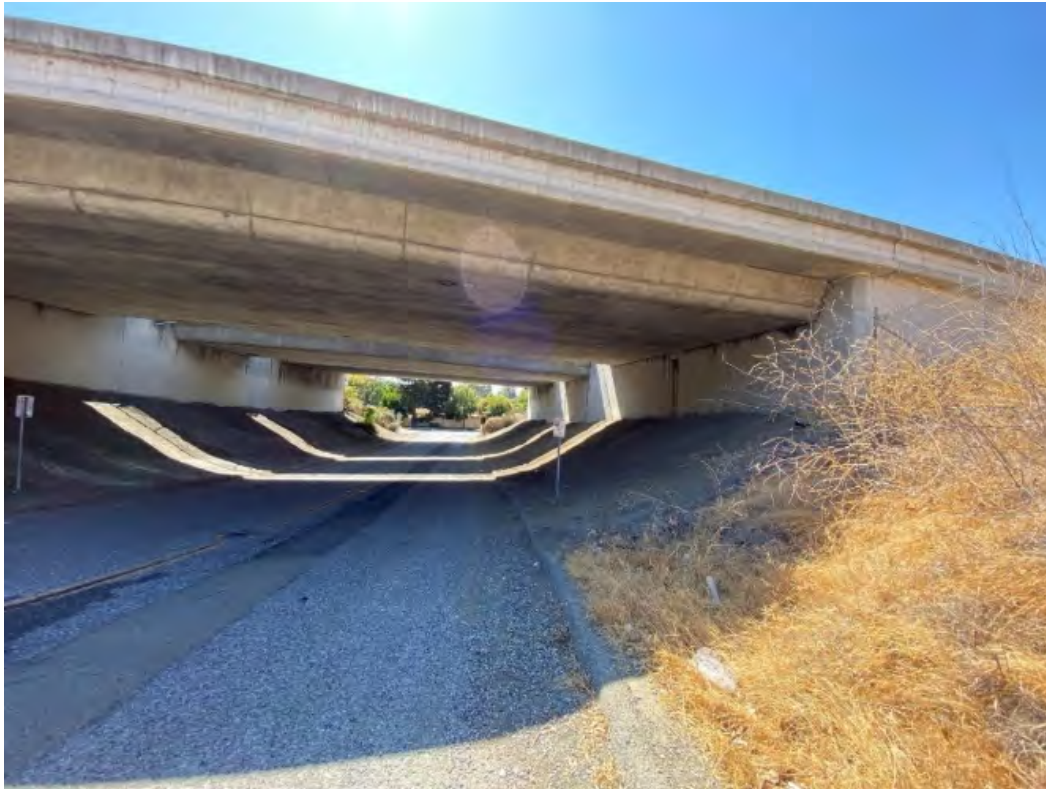
Figure 6: Bicycle and Pedestrian Facilities Missing on Carol Drive between Canoas Garden Avenue and the Highway 87 Bikeway
