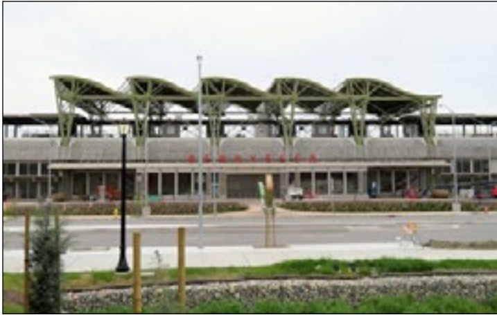
Figure 2.2 Main BART station entrance – view from surface parking lot
