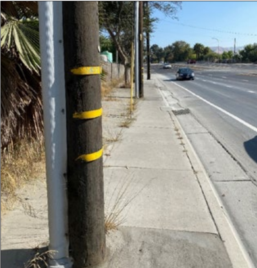
Figure 6.5 Narrow sidewalk on Berryessa Road
