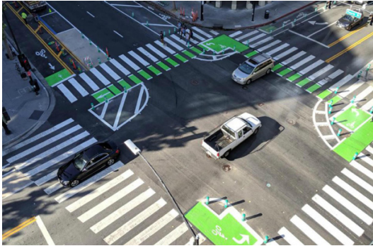
Protected intersection at 4th Street/San Fernando Street intersection.
