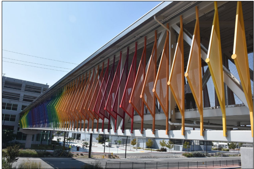
Montague Pedestrian Overcrossing Bridge
