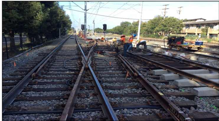
Turnout and switch machine installation near Stevens Creek Bridge
