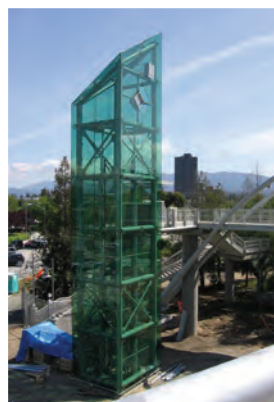
Elevator at the Hamilton Light Rail Station
