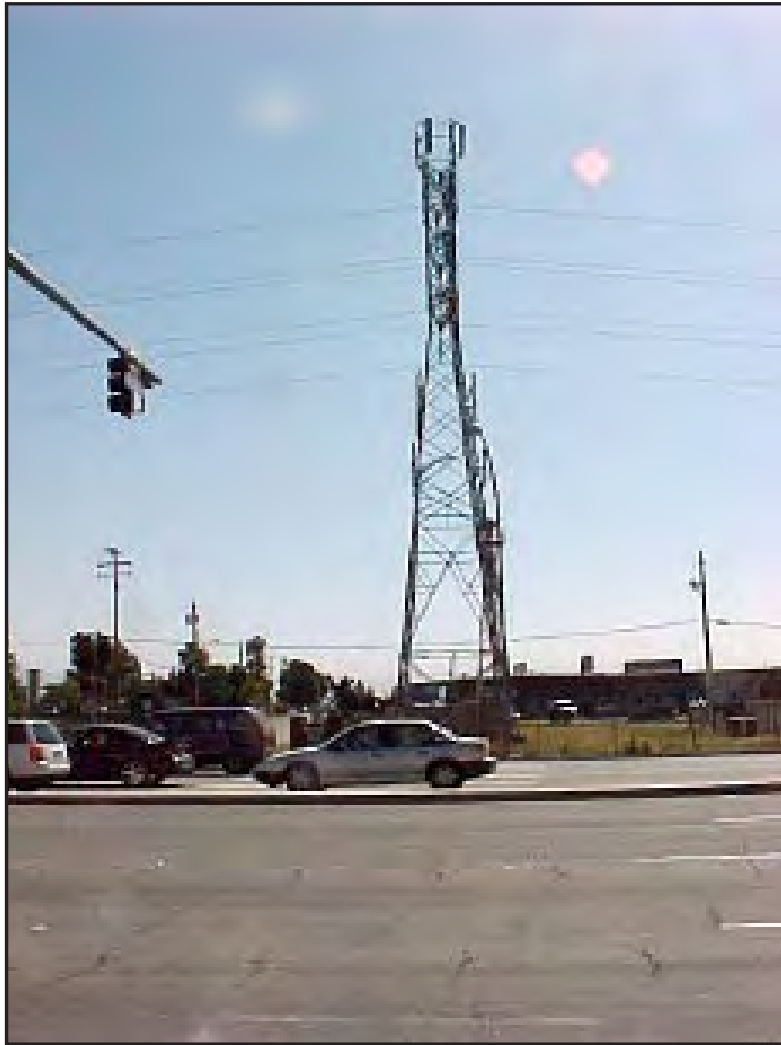
Existing view of electrical transmission tower.
