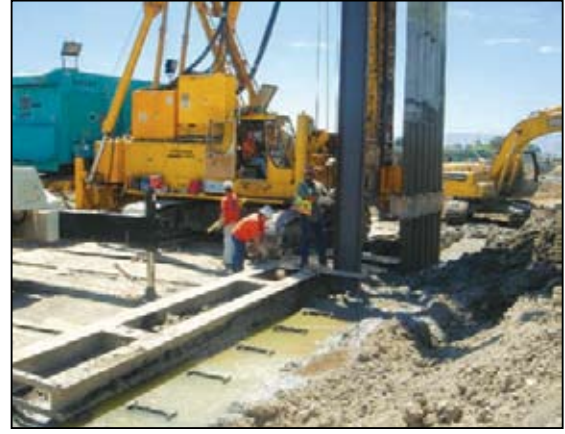
Figure 4.18-6 Deep Soil Mix and Steel Soldier Piles
