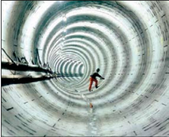
Figure 4.18-13 Example of Segmental Concrete Lining Units and Rings Tunnel Boring Machine
