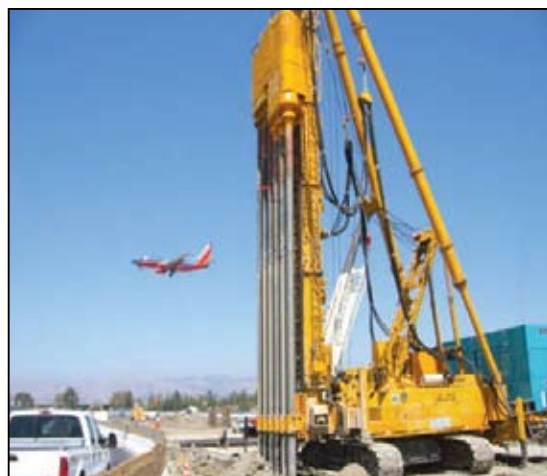
Figure 4.18-5 Deep Soil Mix and Auger Rig Installation
