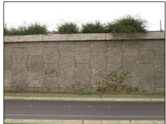
Figure 4.18-19 Mechanically Stabilized Earth Wall
