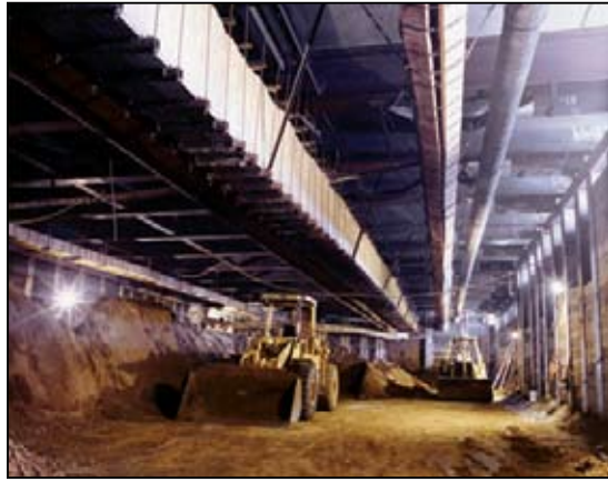
Figure 4.18-4 Temporary Utility Support in an Excavation
