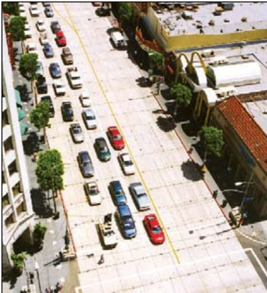
Figure 4.18-2 Temporary Deck Installation
