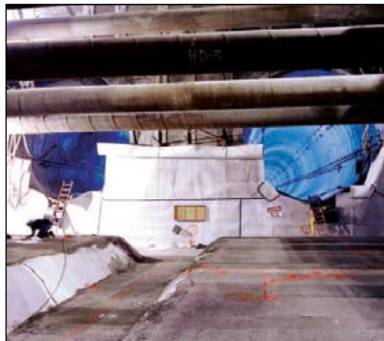
Figure 4.18-23 Lateral-bracing Members
