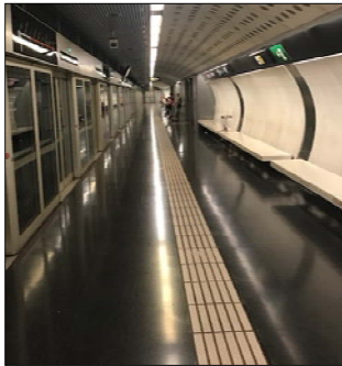
Station platform within the tunnel
