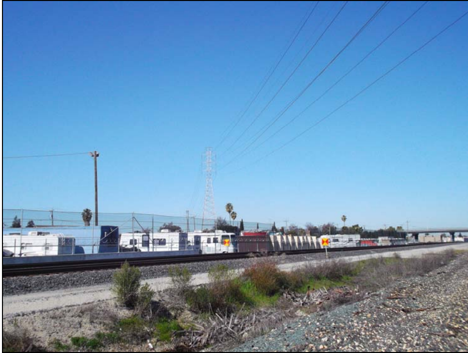
Figure 11: View from BART Corridor Looking Northwest Toward Horner Property and Existing 115-kV PG&E Tower
