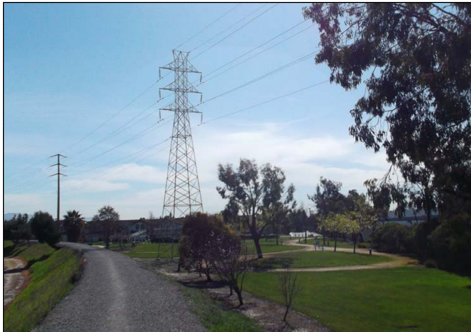
Figure 13: View from Berryessa Creek Levee Looking South Toward Beresford Meadows Park
