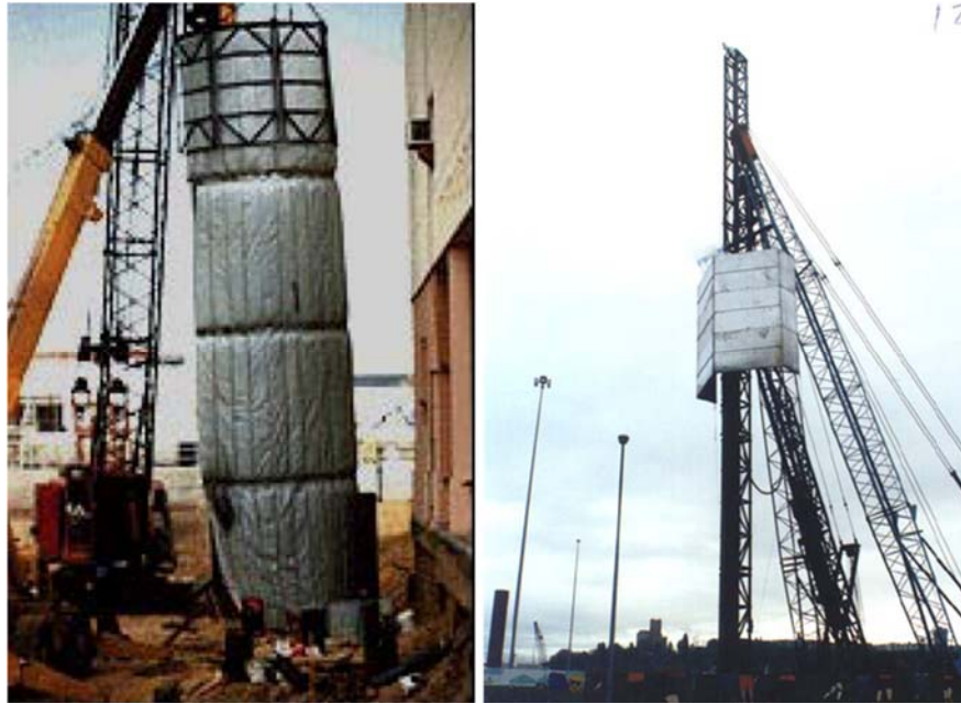
Figure 13: Impact Pile Noise Shrouds. Image on the left shows an effective enclosure. Image on the right shows a marginally effective barrier.
