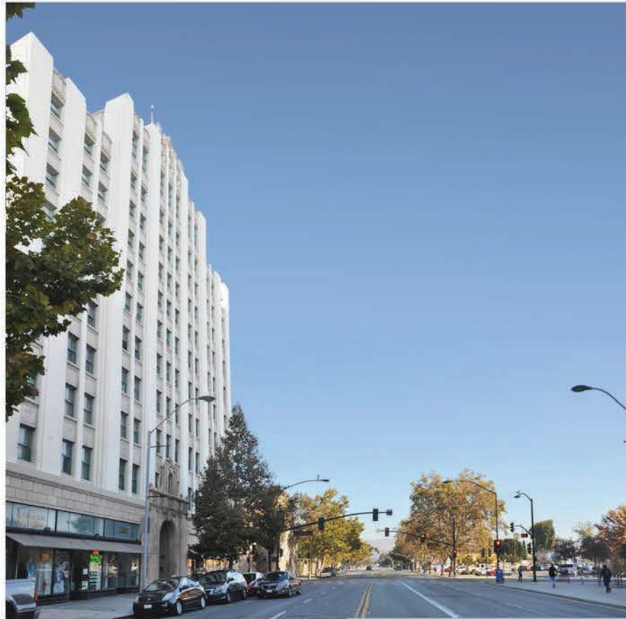
Existing view along Santa Clara Street (view to the northeast from the intersection of East Santa Clara Street and 5th Street)
