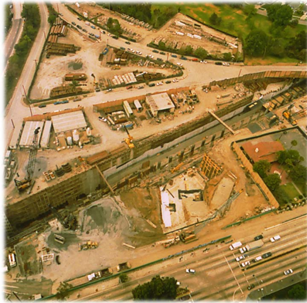
LA Metro – Universal City Station Excavation (similar site constraints as Alum Rock)
