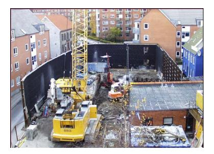
Figure 4.19-29: Construction Site Screening Example #2
