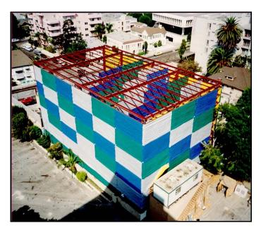
Figure 4.19-28: Construction Site Screening Example #1
