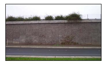
Figure 4.19-3: Example of Mechanically Stabilized Wall
