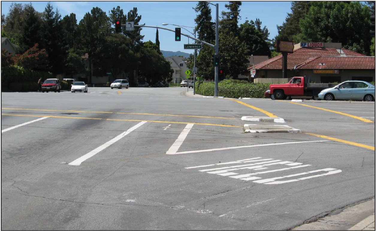
a. View of an example bike slot facing west at Lawrence Expressway and Cabrillo Avenue in the City of Santa Clara.
