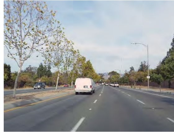
Roadway characteristics include wide lanes, two to seven travel lanes, and slip lanes. These prevalent characteristics along the corridor prioritize vehicle mobility over other modes of travel. Left: Story Road cross section. Below: Willow Street cross section.
