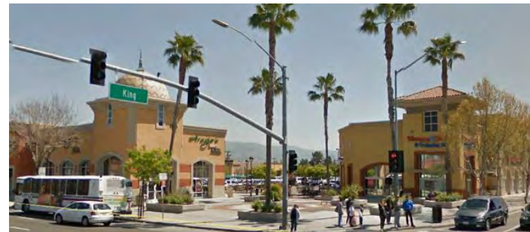
Shopping center along Story Road between King Road and Bal Harbor Way
