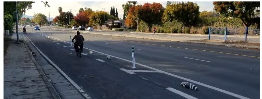
Left: “Paint and plastic” separated bikeways can include striped buffers where parking serves as a barrier between bicycle traffic and auto and transit traffic. Above: The City can use various products to provide separation between the bicycle lane and traffic, including planters and small plastic lumps (sometimes known as “zebras” or “armadillos”), which are already in use on Branham Lane.
