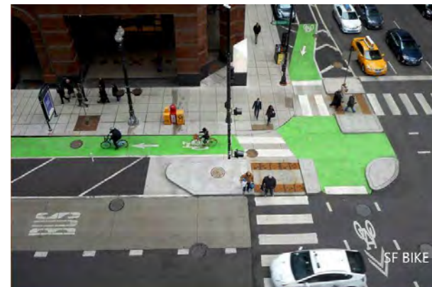
Example of a protected intersection with pedestrian median refuges after the separated bikeway. Source: SF Bicycle Coalition
