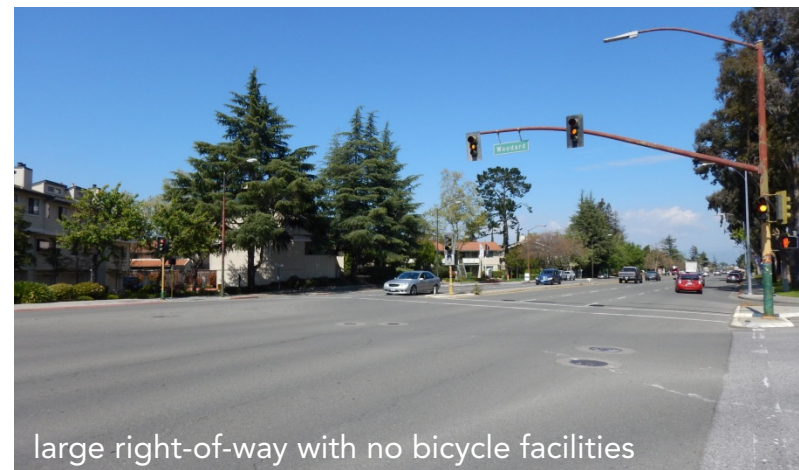
large right-of-way with no bicycle facilities
