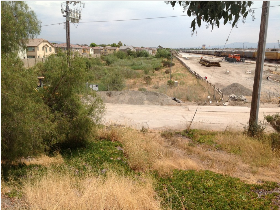
Photo 20. Photo-point 36, looking over the site from the Hwy 237 embankment located north of the site (July 2015)
