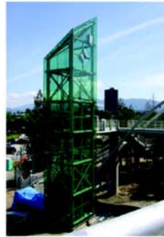
Elevator at the Hamilton Light Rail Station
