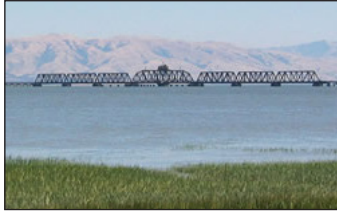
View of Dumbarton Bridge from the west
