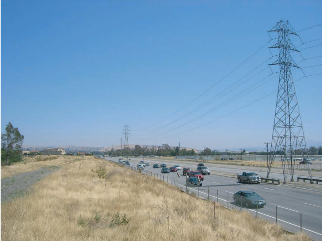
Figure 5-13 Existing View of Capitol Expressway North of Tully Road
