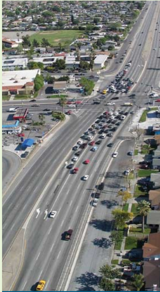
Existing Story Road
