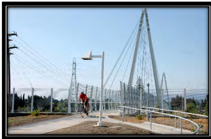
Mary Avenue Bridge
