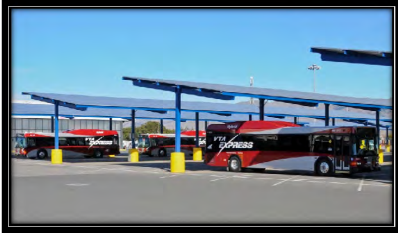
Solar Panels and Express Buses at North Operating Division
