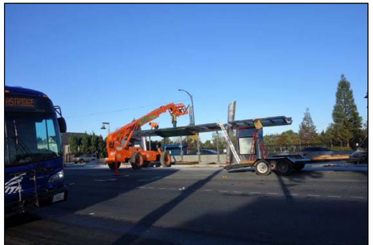
Installation of BRT Station shelter
