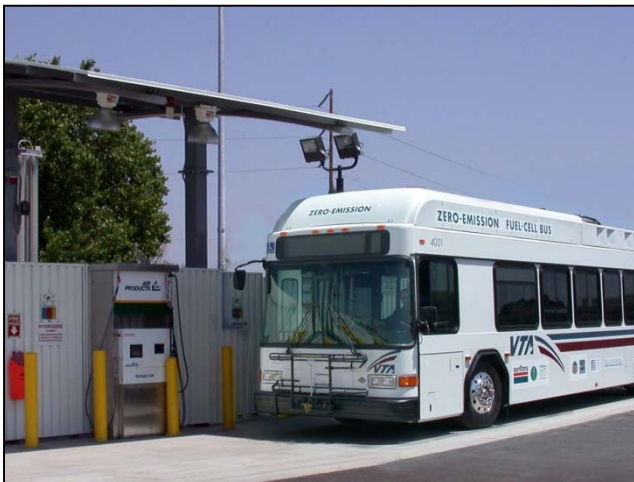
ZEB at Fueling Station
