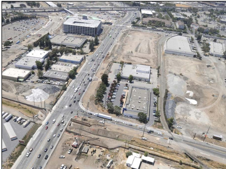
Aerial View of Montague Expressway Reconstruction
