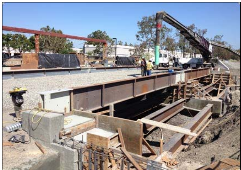
Progress on UPRR Bridge at Kato Road (C222)
