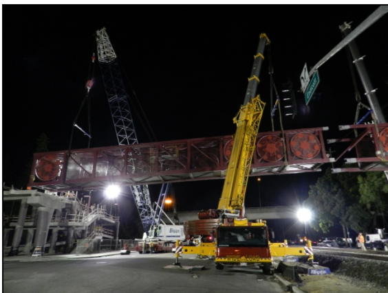
Blossom Hill Pedestrian Bridge Installation
