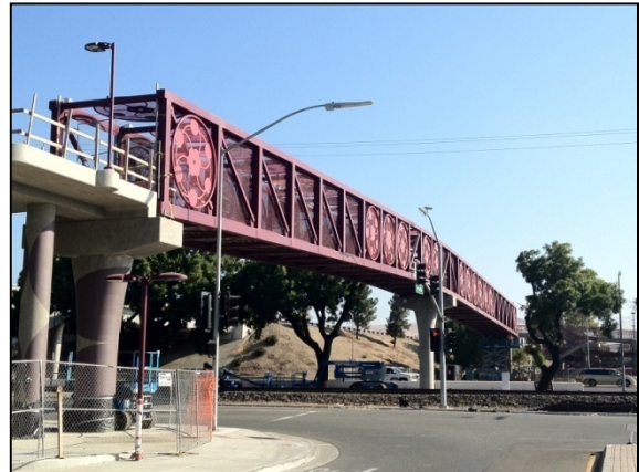
Blossom Hill Pedestrian Bridge Installed
