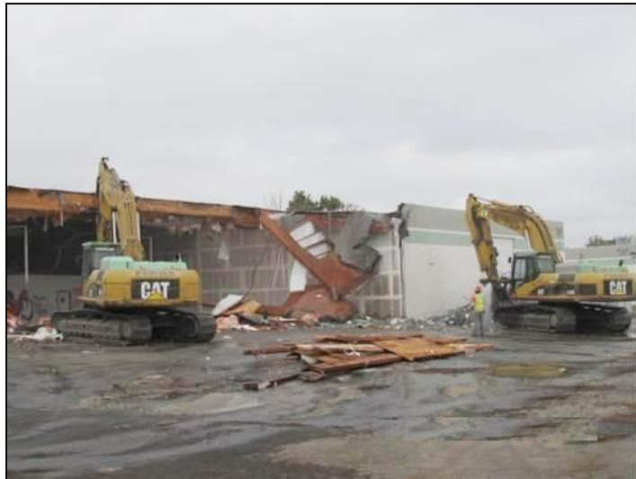
Building Demolition (C700)
