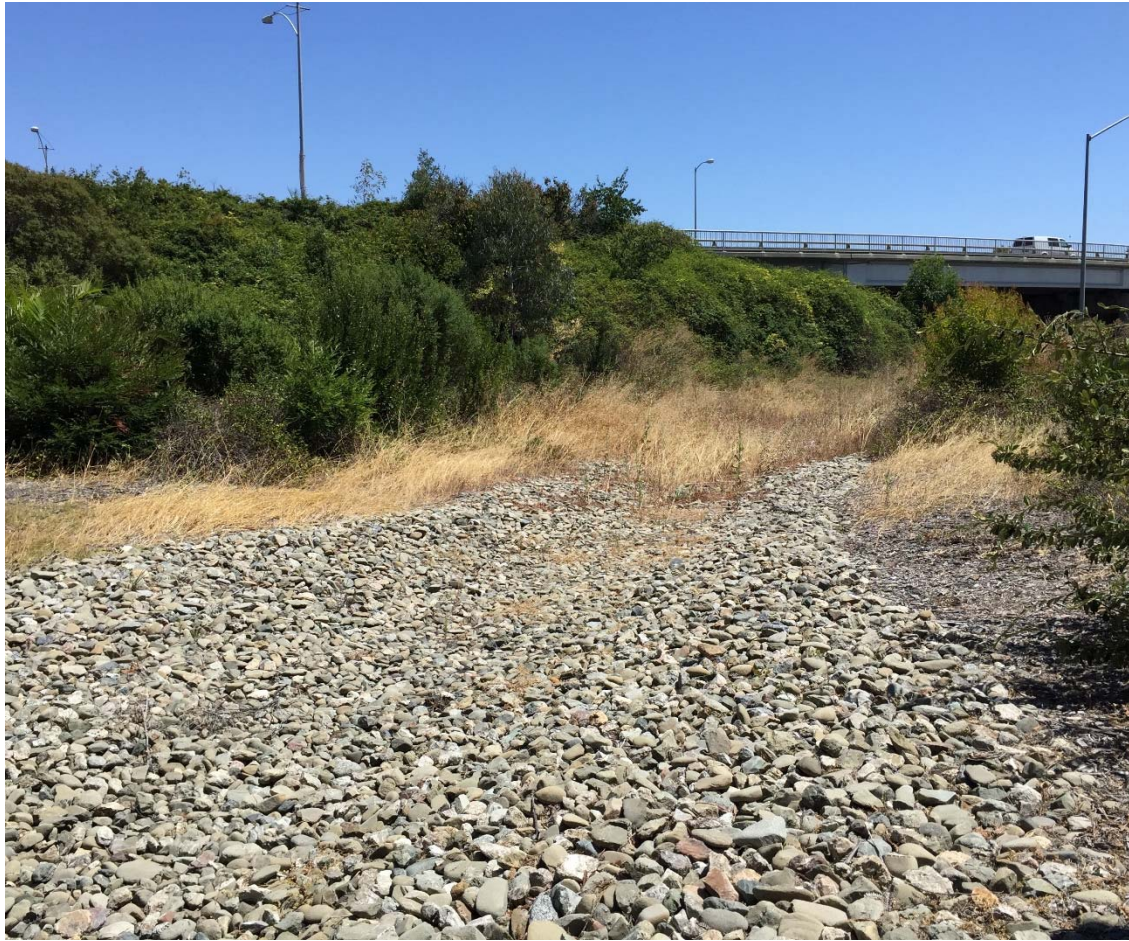
Photo 3. Drainage within US 101 northbound to Mathilda Avenue southbound interchange loop ramp, facing southeast.
