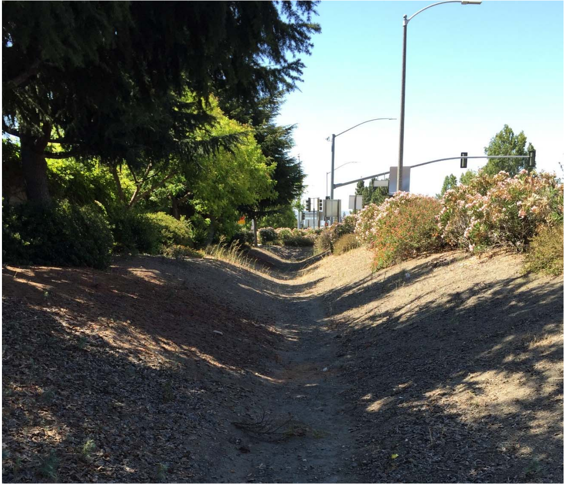
Photo 1. Drainage parallel to Mathilda Avenue, facing south.
