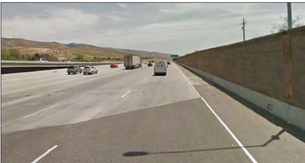
Exhibit D. Southbound US 101 south of SR 85 interchange in southern San Jose, with a sound wall on the west side (right) of the freeway.
