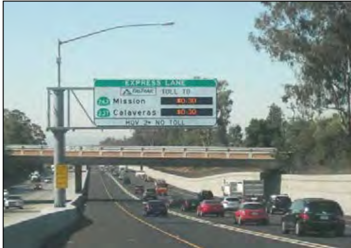
Exhibit M. Representative view of an entrance/toll sign with messaging (from I-680 southbound express lanes in Fremont)
