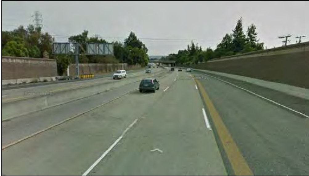
Exhibit L. Southbound SR 85 just south of the SR 85/US 101 interchange in Mountain View, with sound walls and vegetation bordering the freeway
