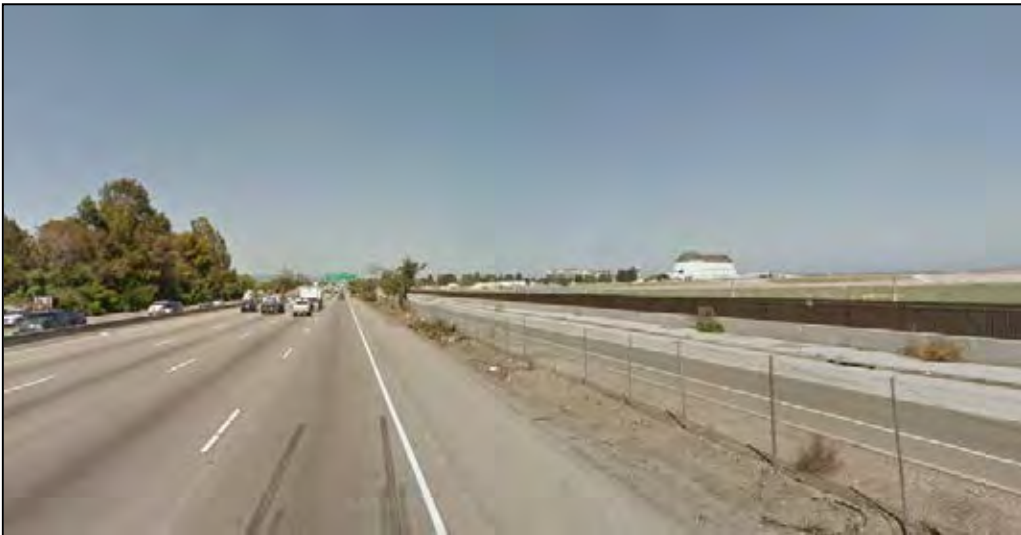
Exhibit J. Northbound US 101 south of Ellis Street interchange near the Sunnyvale/ Mountain View border. Moffett Federal Airfield borders US 101 to the east (right).
