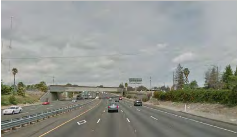
Exhibit H. Northbound US 101 just north of McKee Road in San Jose. A railroad overcrossing and overhead utility lines can be seen in the distance.
