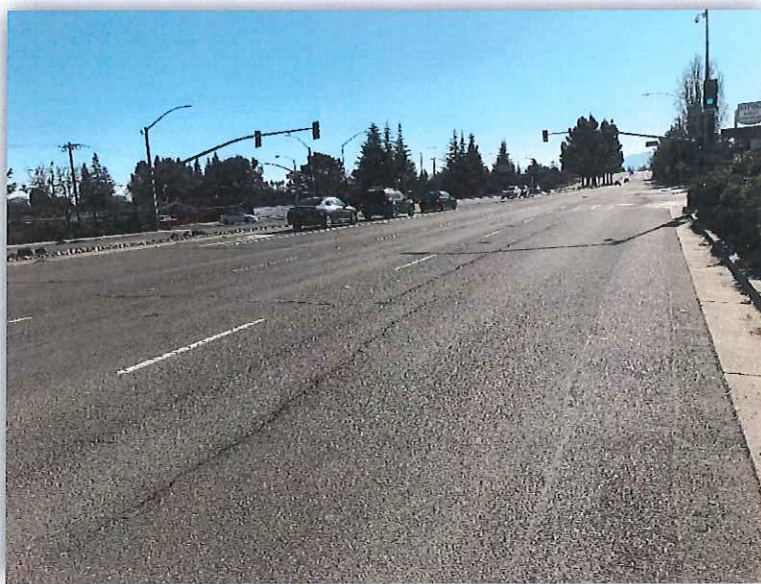
MATHILDA AVENUE – MOFFETT PARK DRIVE TO HIGHWAY 101 NEAR ROSS ROAD (SB)
