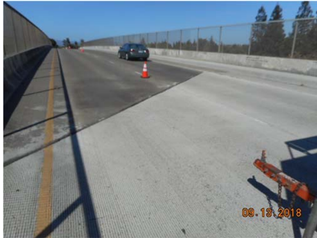
Photo 4 – Typical bridge approach
