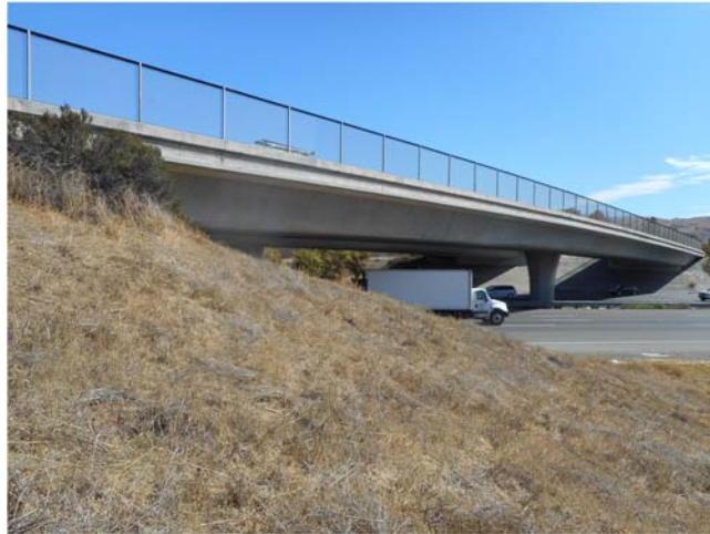
Photo 1 – Blossom Hill Road OC (37-0348L/R) in Santa Clara County, California
