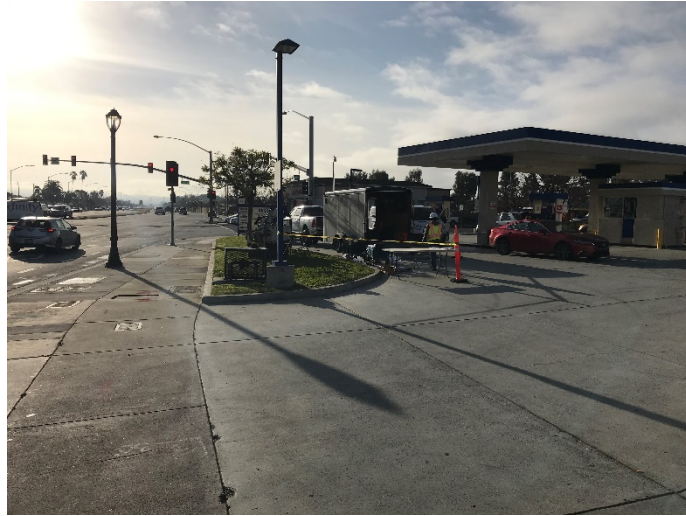
Photo 1: View of drilling operation and safety zone (facing south).
