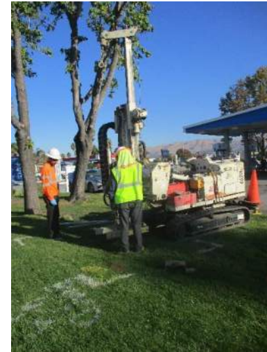
Photo 6: Direct Push Drilling.
