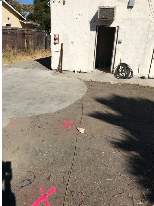
Photo 3: View of potential site of monitoring well (MW-7) installed in 1987 to 25 feet below ground surface (bgs) and destroyed in 2010 by WDC Exploration and Wells and inspected and approved by the Santa Clara Valley Water District (SCVWD) (facing east).
