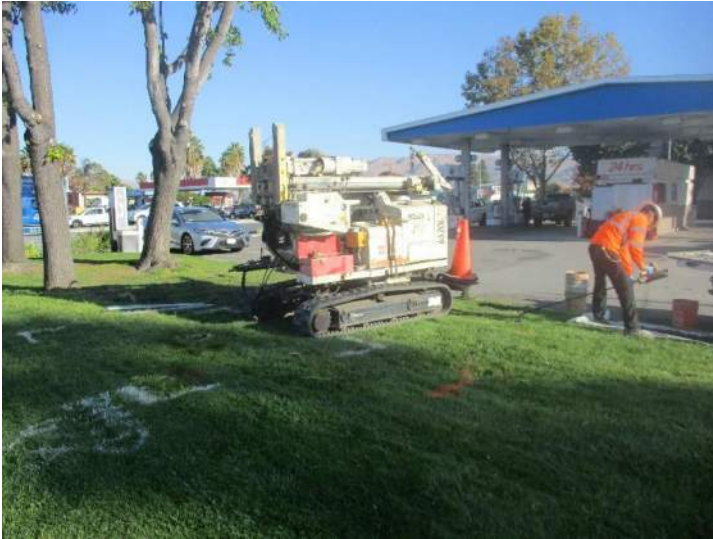
Photo 5: Hand Clearance of boring.
