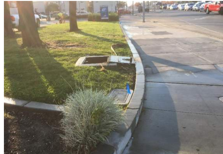
Photo 2: Pressure grouted groundwater extraction well.
