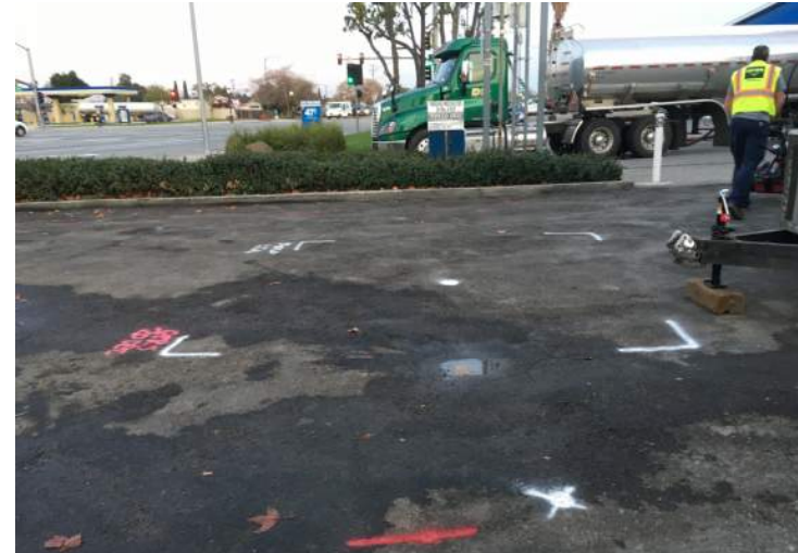
Photo 2: Boring B-2 relocated to the right due to subsurface electric line.
