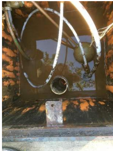
Photo 3: Former Groundwater extraction well.; Pressure Grouted.
