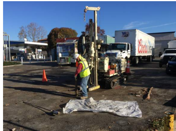
Photo 4: Hand clearance and GeoProbe (B-1).
