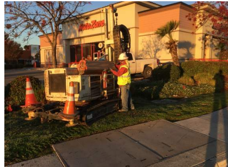
Photo 4: Direct Push Drilling (B-1).
