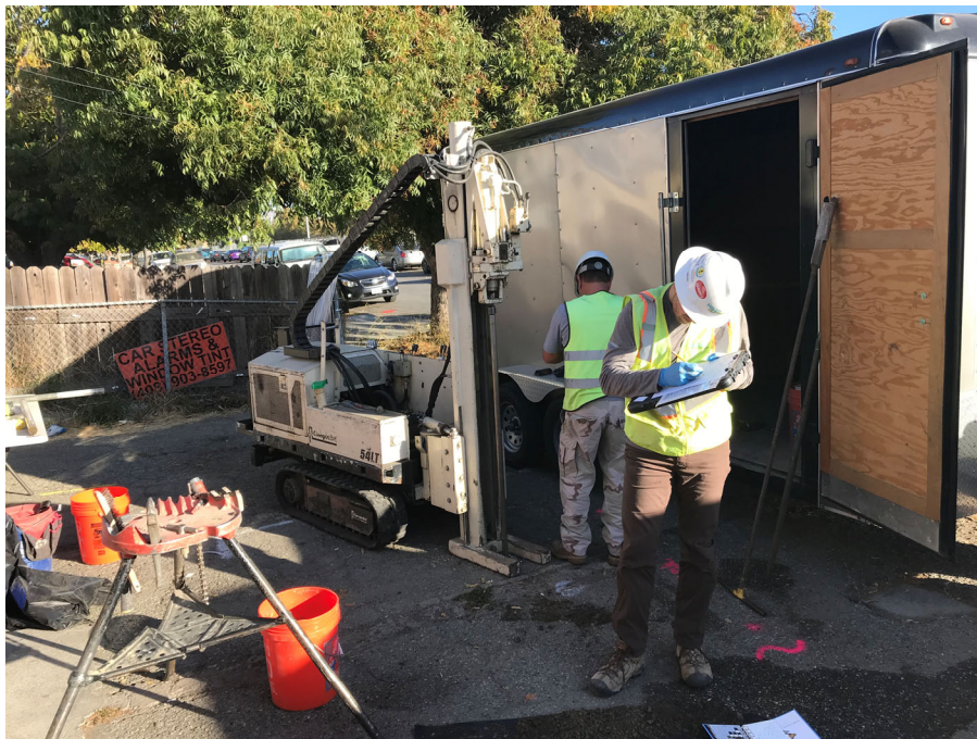
Photo 4: View of drilling at SB-1 (facing north).
