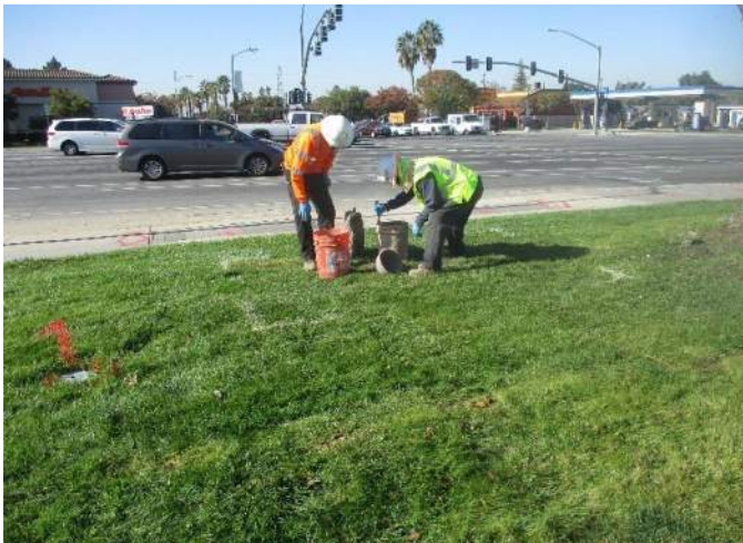
Photo 7: Boring backfilling.
