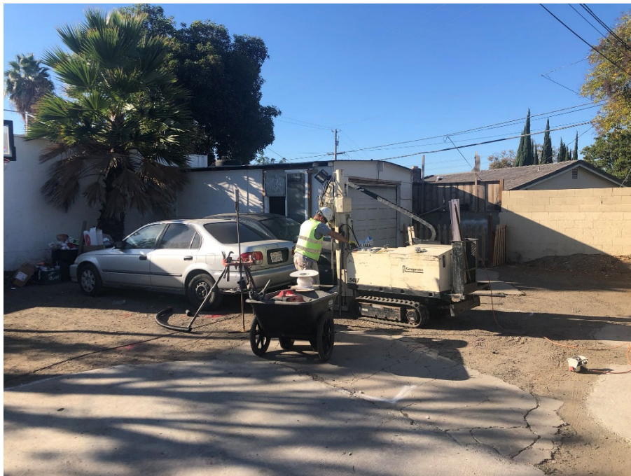
Photo 6: View of drilling at SB-2 (facing west).
