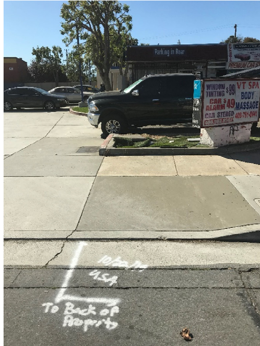
Photo 1: View of USA markings and front of property (facing west).
