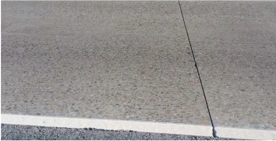
Location ST-55 in the proximity of Sea Gull Court, Saratoga
