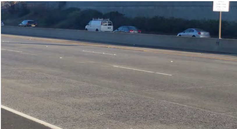
Location ST-24, in the proximity of The Dalles, Sunnyvale
