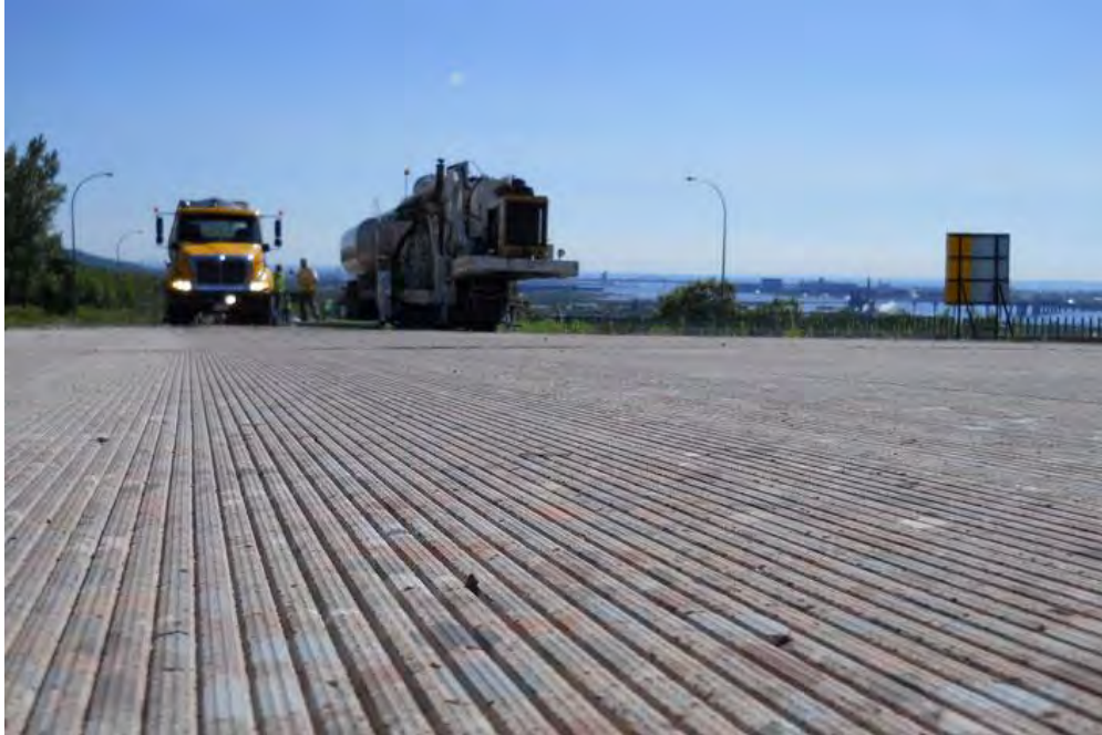
Figure 5-9: Next Generation Concrete Surface (NGCS) Grind and Groove (GnG) pavement.
