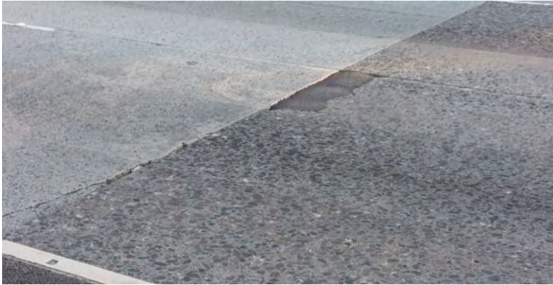
Location ST-19, in the proximity of Lubich Drive, Mountain View
