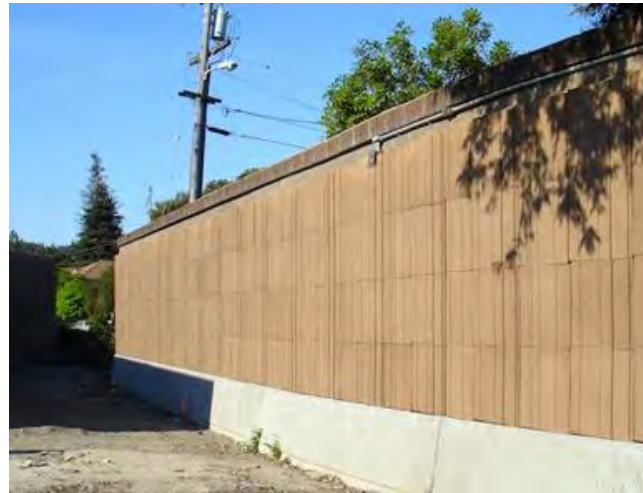
Figure 5-5: Acoustically Absorptive Barrier Tiles
