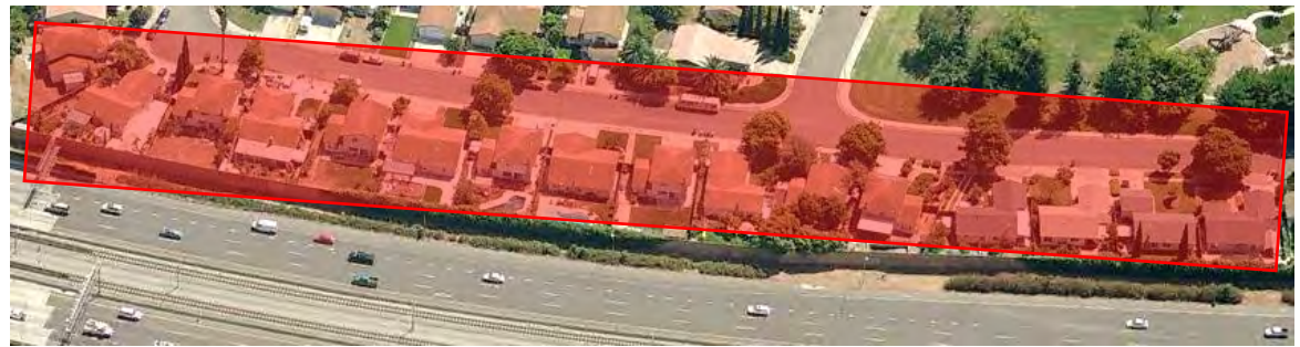
Bird's Eye View Looking West
