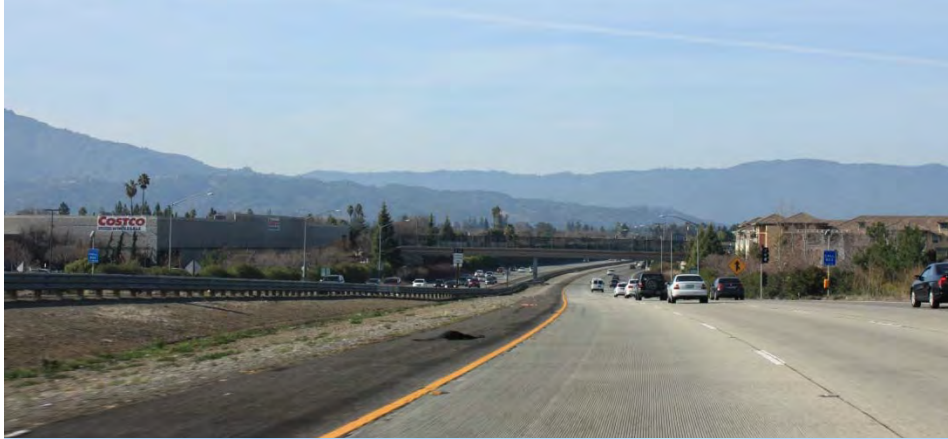
Exhibit B. Elevated section of SR 85, northbound direction, viewed from just west of Almaden Expressway interchange in San Jose.
