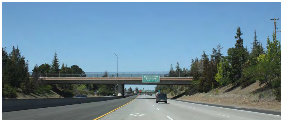
Exhibit I. Northbound SR 85 in Cupertino, at McClellan Road overcrossing approaching Stevens Creek Boulevard.
