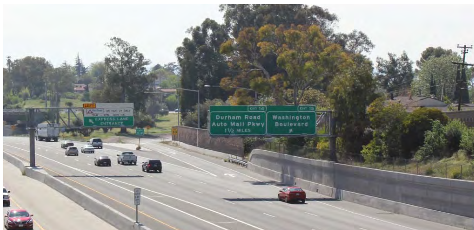
Exhibit V. A second perspective of the representative view of the I-680 southbound express lanes in Fremont. This photo shows the same median-mounted express lane sign (green and white) in the context of other similar size and height directional freeway information and exit signs (all green).
