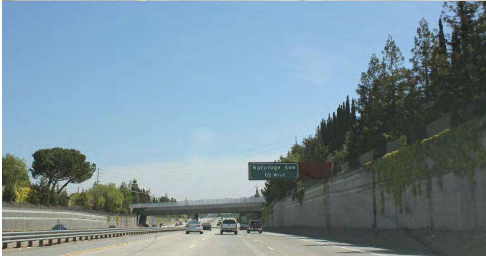
Exhibit G. Southbound SR 85 in Saratoga just north of Cox Avenue underpass, approaching Saratoga Avenue exit.
