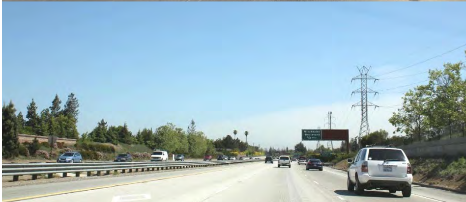
Exhibit D. Southbound SR 85 in Los Gatos, approaching Winchester Boulevard. Freeway has landscaped side slopes on both sides, bordered by sound walls. Transmission line corridor on right side of right-of-way.
