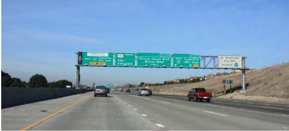
Exhibit L. Northbound US 101 south of SR 85 interchange in southern San Jose, with a gantry (a structure that spans the roadway and is supported by posts on both sides) in the foreground and residential development to the east (center and right side of photo).
