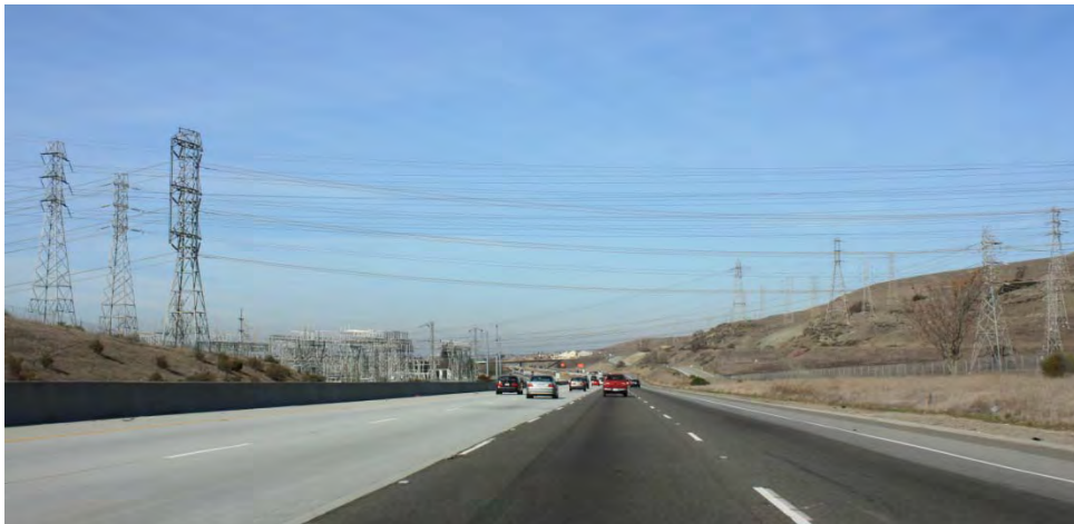
Exhibit K. Northbound US 101 north of Bailey Avenue in southern San Jose. The PG&E Metcalf Substation is just west (left) of the southbound lanes.
