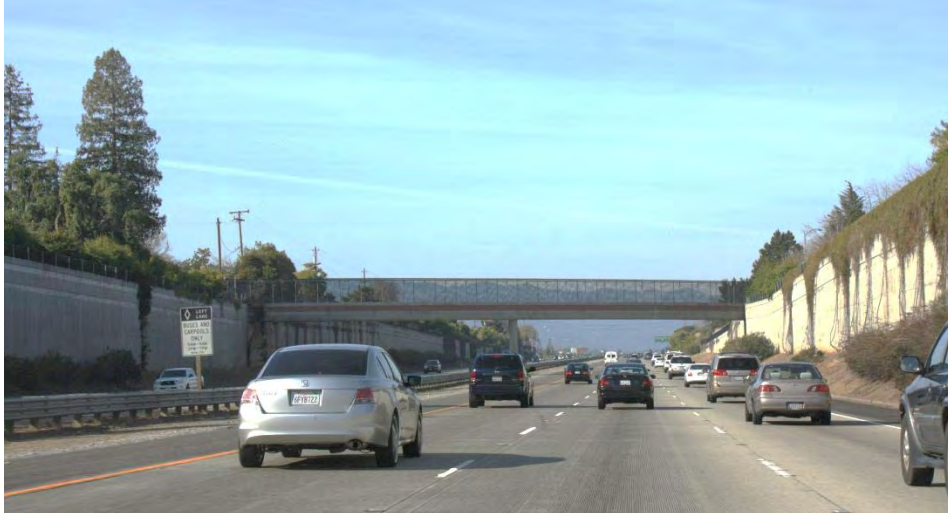
Exhibit C. Depressed section of SR 85, viewed from northbound SR 85 west of Camden Avenue in San Jose.
