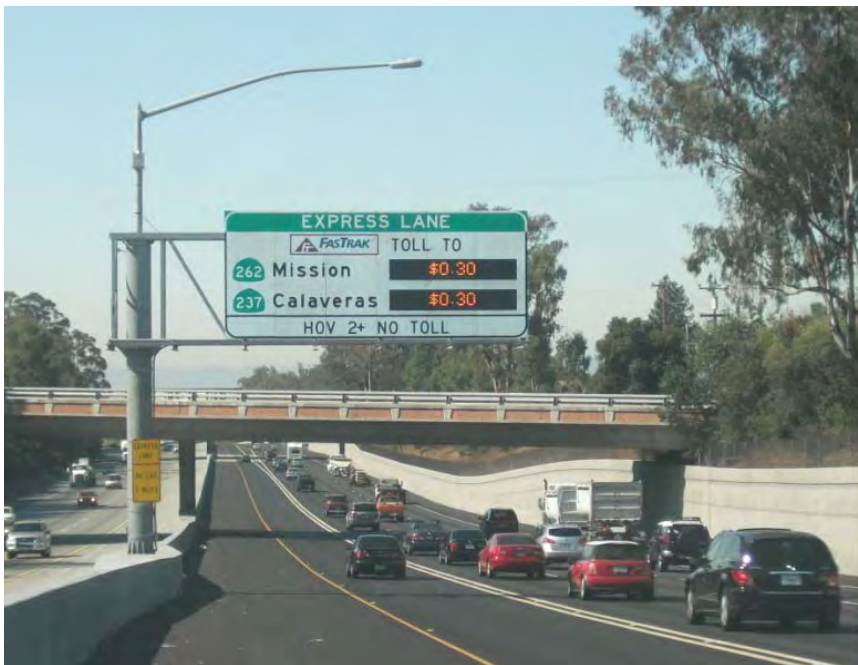
Exhibit R. Representative view of an entrance/toll sign with DMS and mast-arm luminaire (from I-680 southbound express lanes in Fremont).
